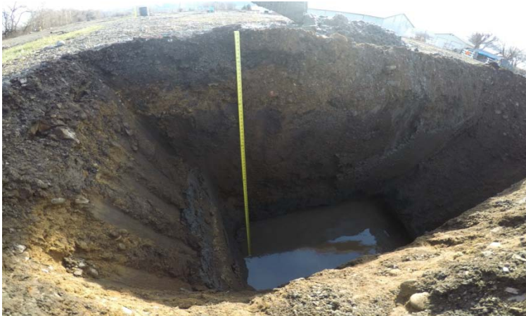
Typical test pit advanced to approximately 8 feet bgs. Depth to groundwater in this pit is approximately 7 feet bgs.
