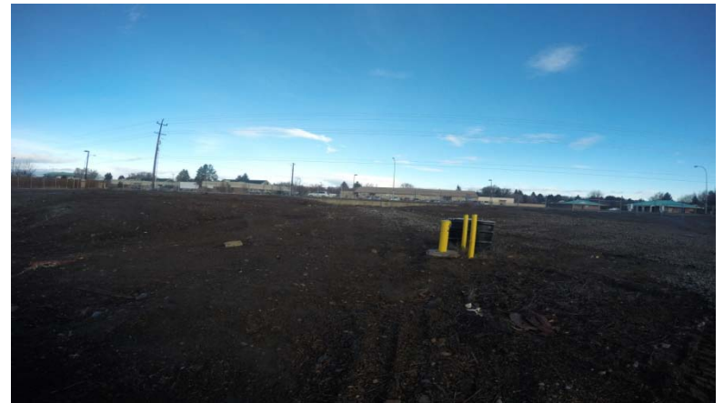
In this photo a groundwater monitoring well can be seen. All but one monitoring well at the site was constructed like this.
