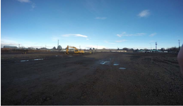
Site facing north.
