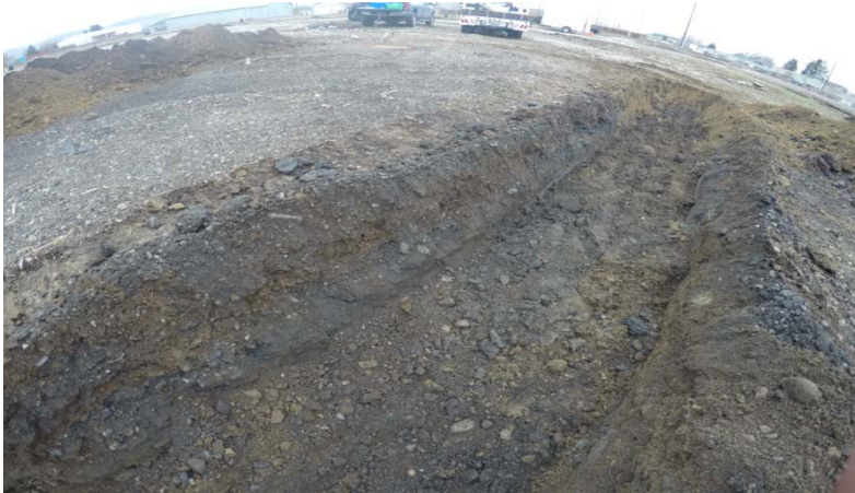
This is a photo of a trench dug for surface sampling. Variable coloration changes can be seen throughout the trench.
