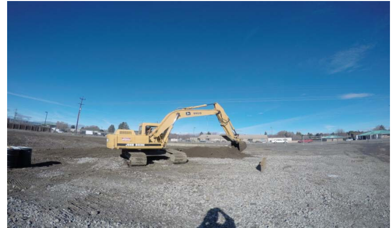
Test pitting on February 10, 2015.
