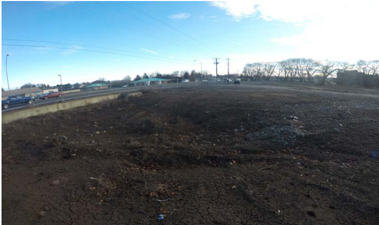
Site facing east near the former scales. Concrete foundation on the left is part of the former scale.
