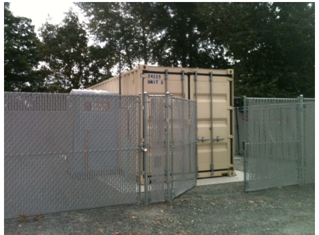
Photograph 16. Example of the remediation system conex housing on the TOC/Farmasonis Property.
