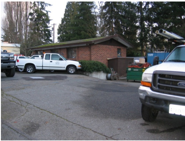
Photograph 1. View of the former building on the TOC Property, looking northeast from 56 th Avenue West.
