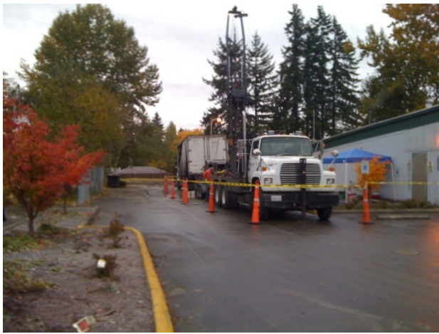
Photograph 13. Hollow-stem auger drill rig and support truck on the Drake Property.
