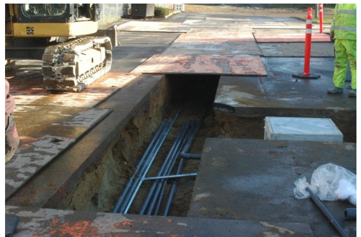
Photograph 14. Remediation system piping installed in a trench on the Drake Property.
