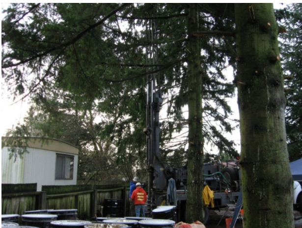
Photograph 11. Hollow-stem auger drilling with a limited-access rig on the TOC Property.
