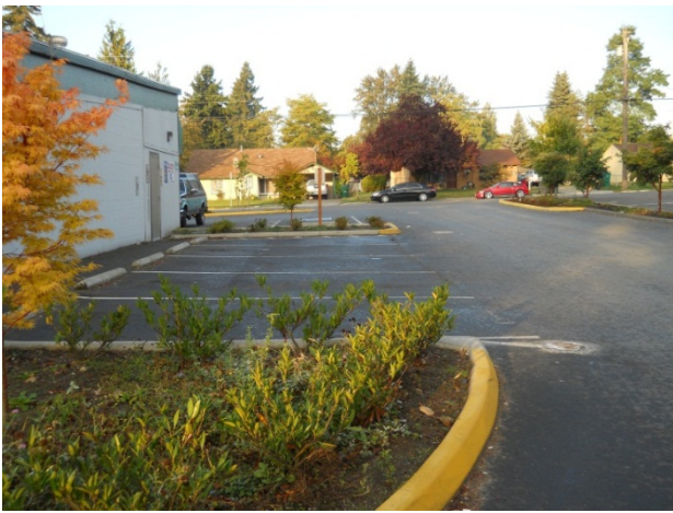
Photograph 7. Northern side of the building on the Drake Property, facing west.
