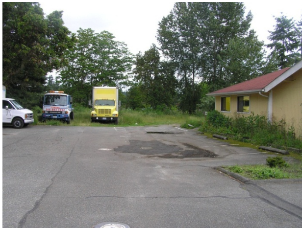
Photograph 5. Portions of the parking lot and grass-covered back lot of the TOC/Farmasonis Property, looking east.
