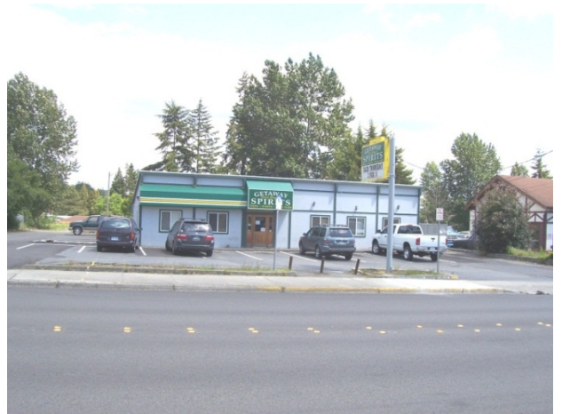
Photograph 6. Front of the Drake Property, looking east across 56 th Avenue West.
