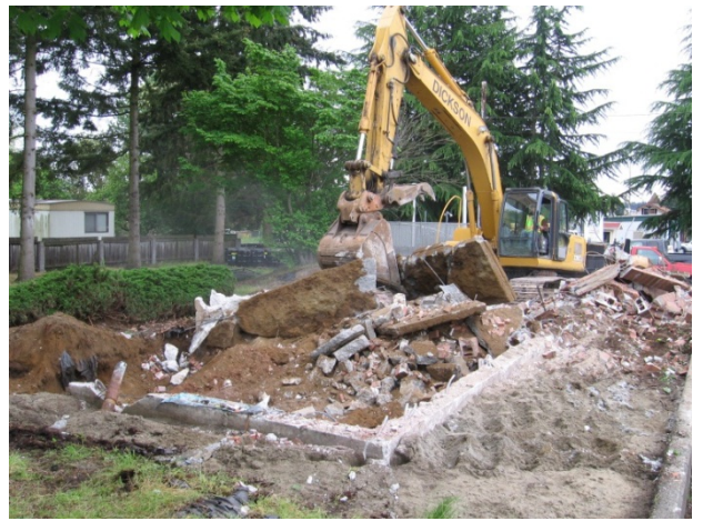
Photograph 2. Demolition of the former building on the TOC Property.
