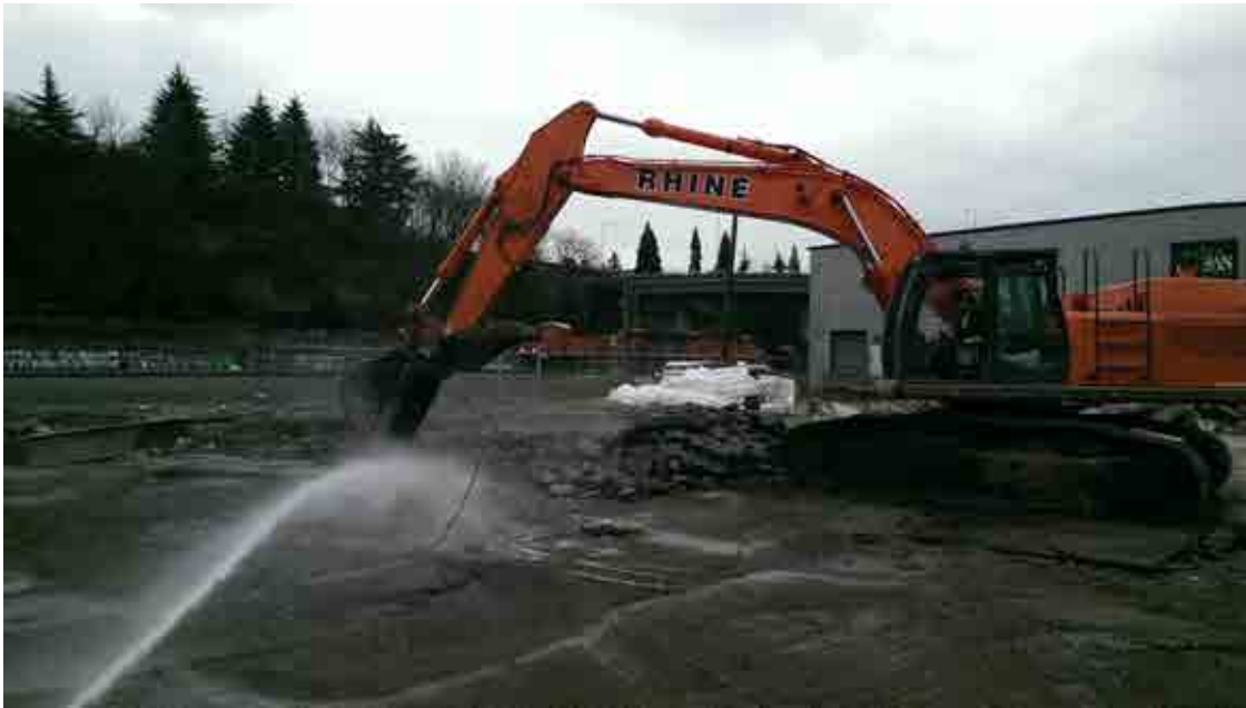
Photograph 1 Concrete slab removal.
