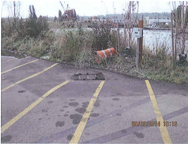
#5. DESCRIPTION: This catch basin has been upgraded to include a large vault that intercepts stormwater and pumps to the treatment system seen in photo # 4. Used to an outfall location.
