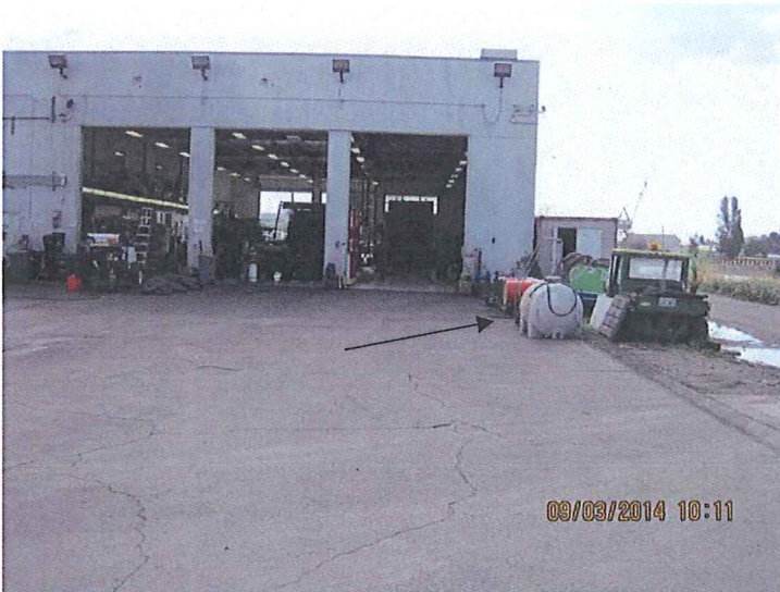
#3. DESCRIPTION: Drums and containers of maintenance fluids (see arrow) are stored along the edge of the bermed area. The facility must ensure that a leak or release will not flow to the storm drainage system.
