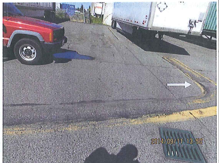
#12. DESCRIPTION: Asphalt berm surrounding fuel island. White arrow indicates cut in berm.
