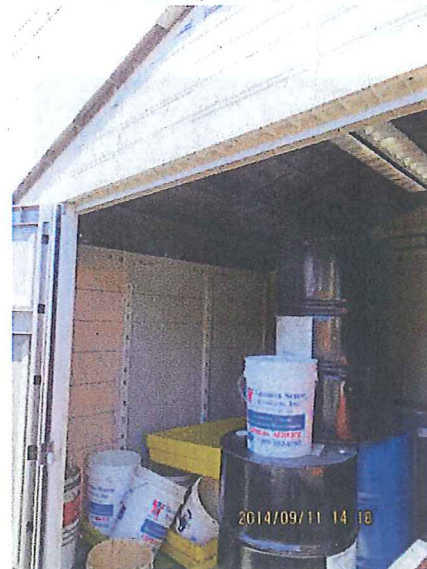
#8. DESCRIPTION: Storage of petroleum product/waste containers in the Waste Oil Shed.
