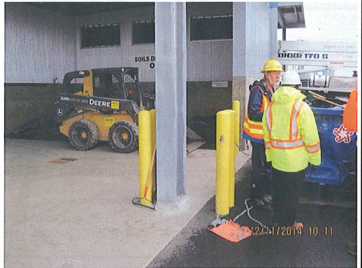
04 DESCRIPTION: DECANT SOLIDS LOADED FROM CONCRETE DRYING AREA (SANITARY) TO BLUE STORAGE BIN ON ASPHALT (STORM).
