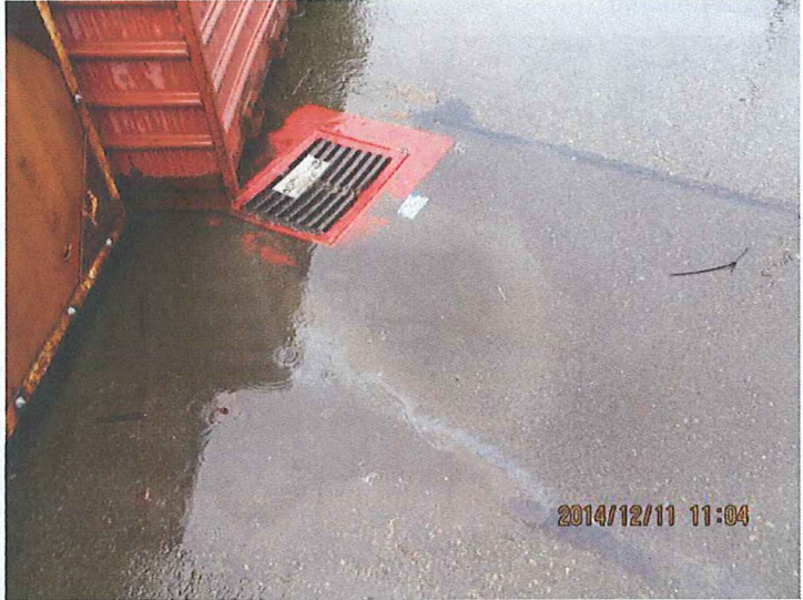
08 DESCRIPTION: CATCH BASIN IN SCRAP YARD. SHEEN.
