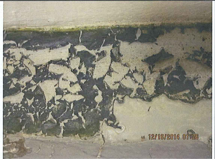
14 DESCRIPTION: DRIED ALGAE IN SEEP DRAIN CHANNEL
