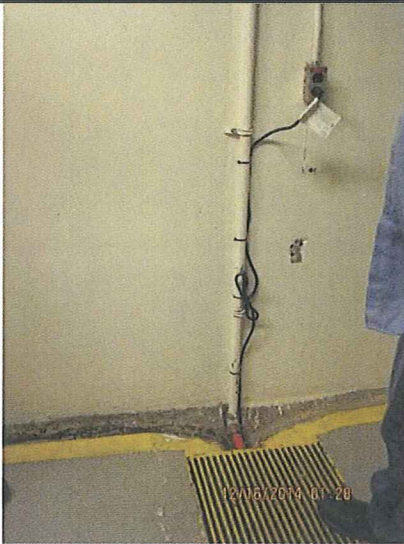
13 DESCRIPTION: CONTROL HOUSE BASEMENT SECONDARY SUMP PUMP
