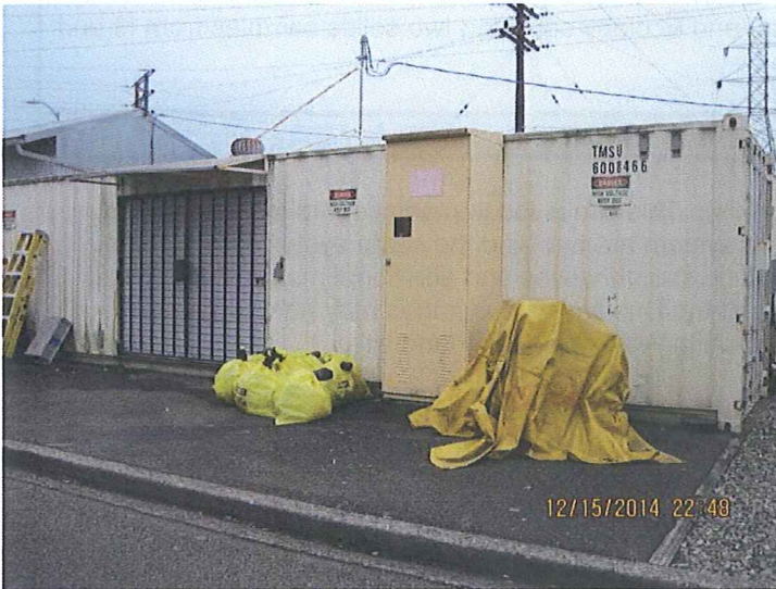
01 DESCRIPTION: MATERIALS STORAGE
