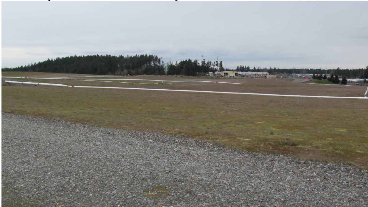
Photo 2: Cap Surface with Gas Collection System – from the east
