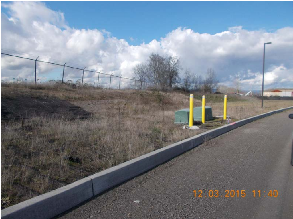
Photo 5: Former Dike Underground Storage Tanks
