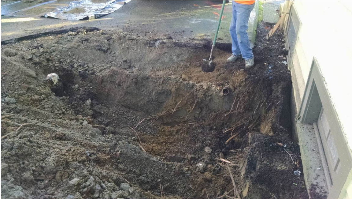
Photograph 4 – Beginning excavation at east 'cell.' Surficial soils and 2007 backfill removed and segregated. 4-inch PVC well casing visible to left of photograph.
