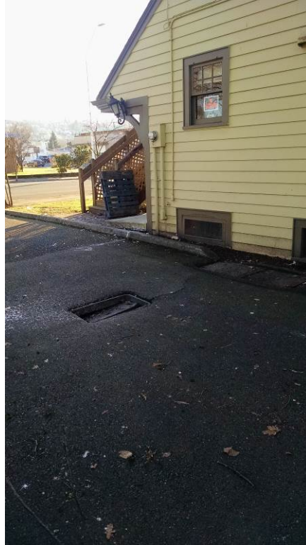
Photographs 1&2 – Area of remedial excavation prior to asphalt removal. Approximate planned extent of excavation marked on pavement. Utility cover protects 4-inch monitoring/dewatering well installed by Riley (2007).
