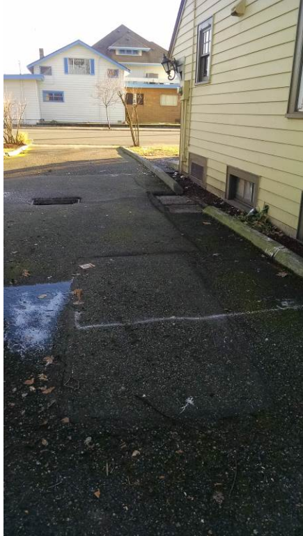
Photographs 1&2 – Area of remedial excavation prior to asphalt removal. Approximate planned extent of excavation marked on pavement. Utility cover protects 4-inch monitoring/dewatering well installed by Riley (2007).
