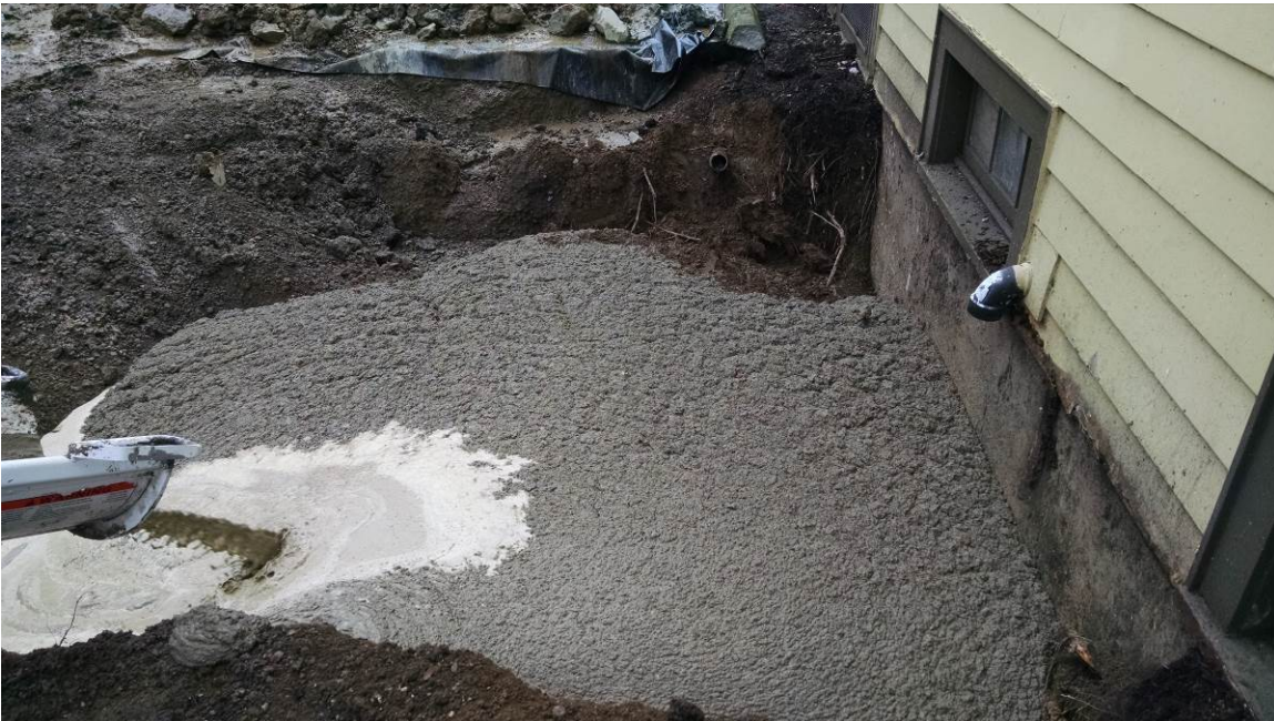
Photograph 7 – Backfilling central 'cell' after completion of remedial excavation on January 15, 2015.
