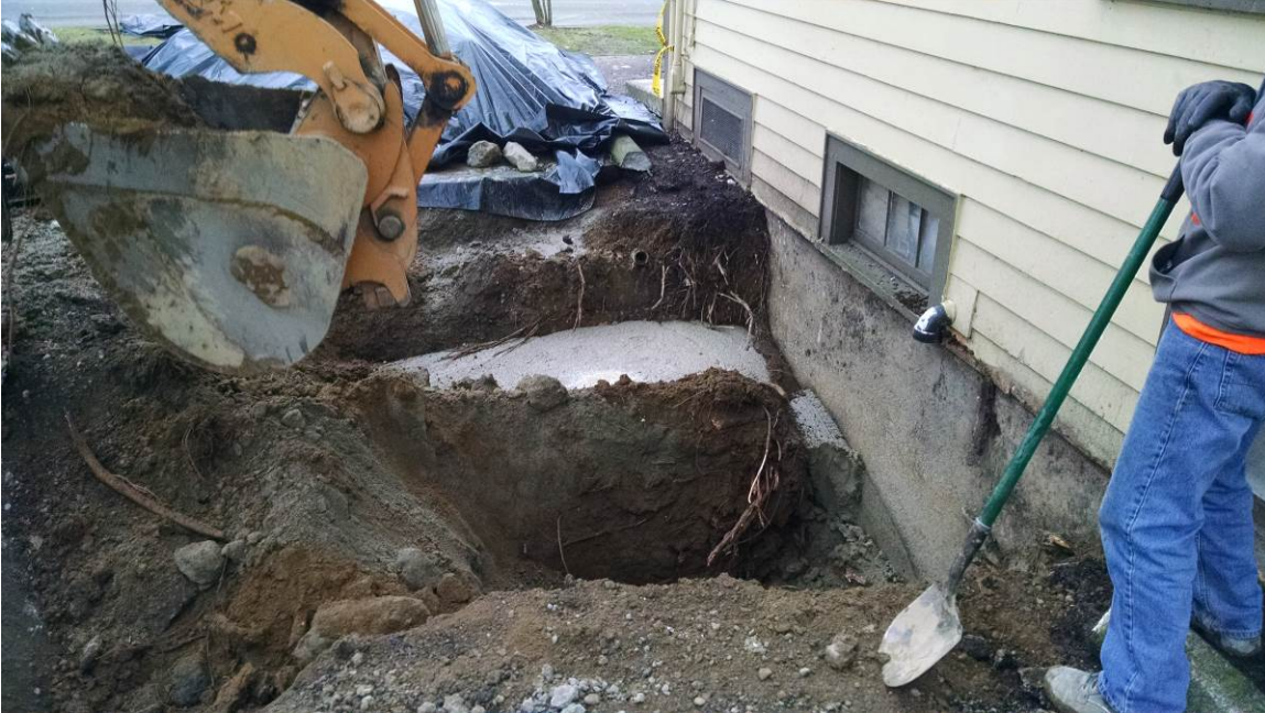
Photograph 6 – East and west 'cells' backfilled with CDF to stabilize excavation, January 13, 2015.
