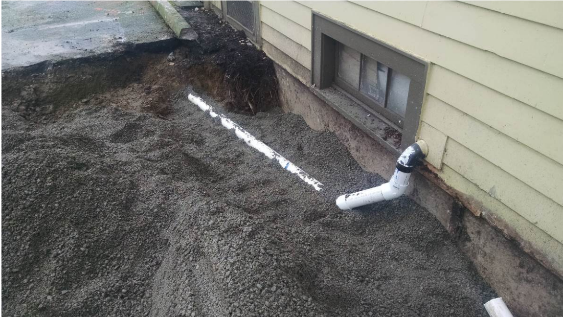
Photograph 8 – Surfacial backfill and sewer line replacement, January 16, 2015
