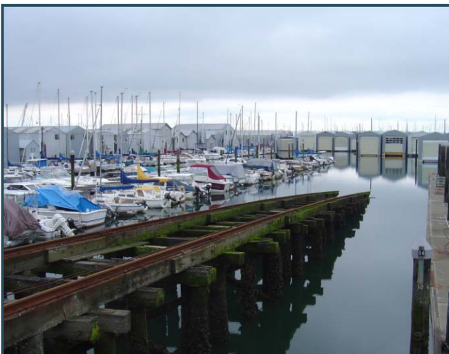
The Marine Railway at the Everett Shipyard, Inc. Site, which was used to move boats from the water to the shipyard for repair.
