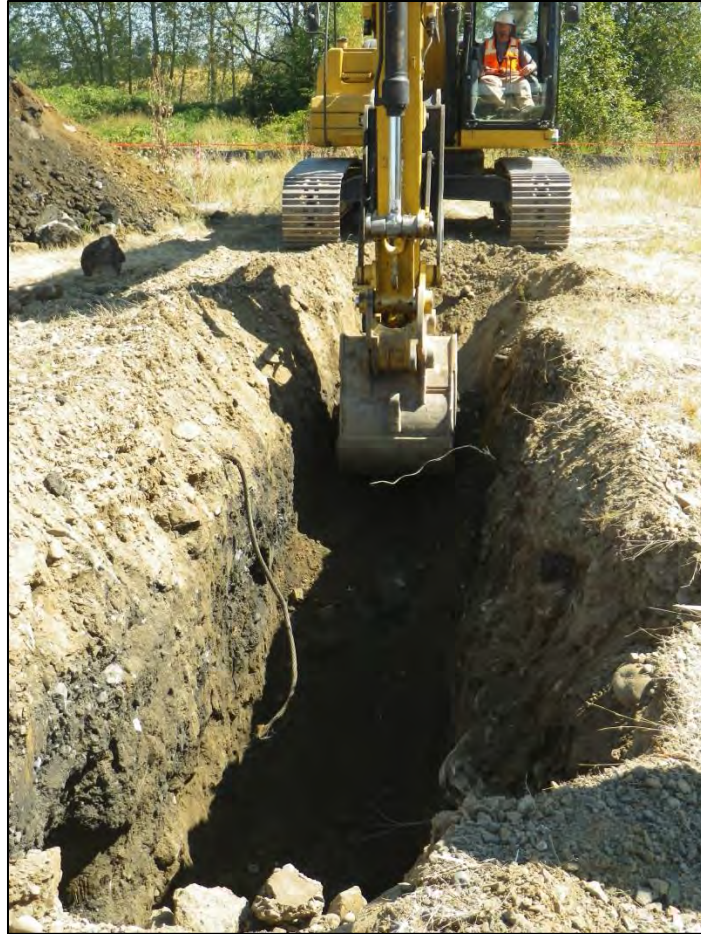
Figure 5. C-2 in progress, fill deposits and top of native sediment visible in trench wall and base of excavation. View to northeast.
