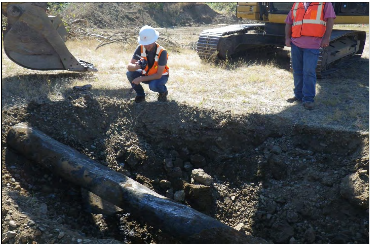
Figure 4. Steel bollard within fill deposits in C-1, view to southeast.
