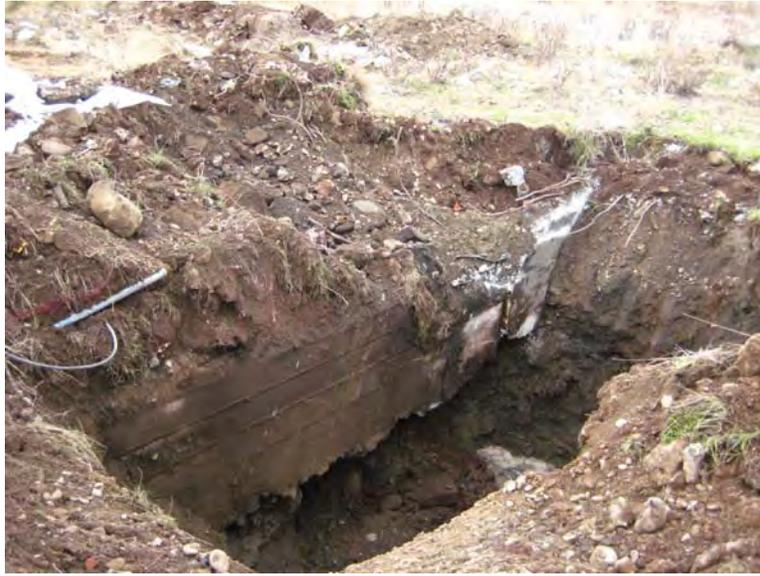
Figure 11. Concrete footer/foundation wall in TP-1.
