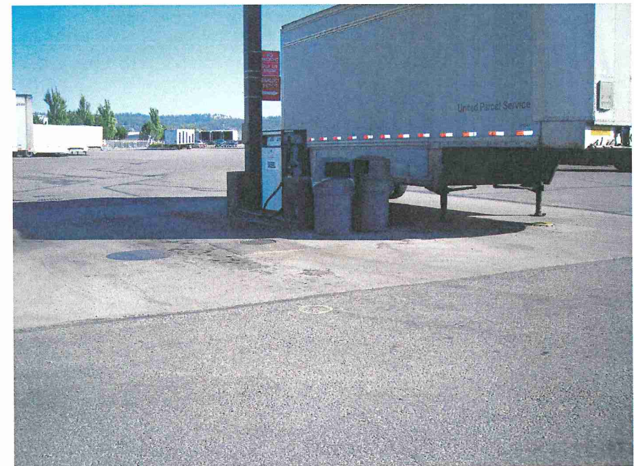
Photograph No. 6: View of the active diesel UST/dispenser area with a proposed boring location (chalk circle) in the center of the photograph.
