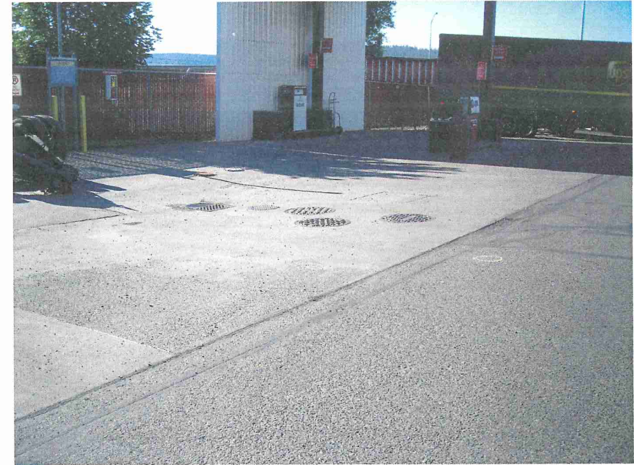
Photograph No. 5: View of the active gasoline UST/dispenser area with a proposed boring location (chalk circle) in the right center of the photograph.
