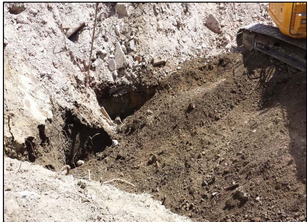
Petroleum-impacted overburden soil stockpile backfilled in UST excavation – looking southeast
