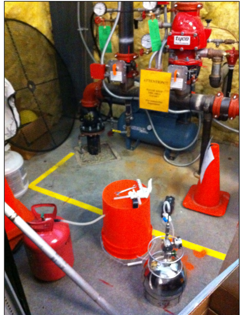
14. Sub-slab soil vapor (i.e. soil gas) sample SSV45 at Junior Achievement collected in storage room.
