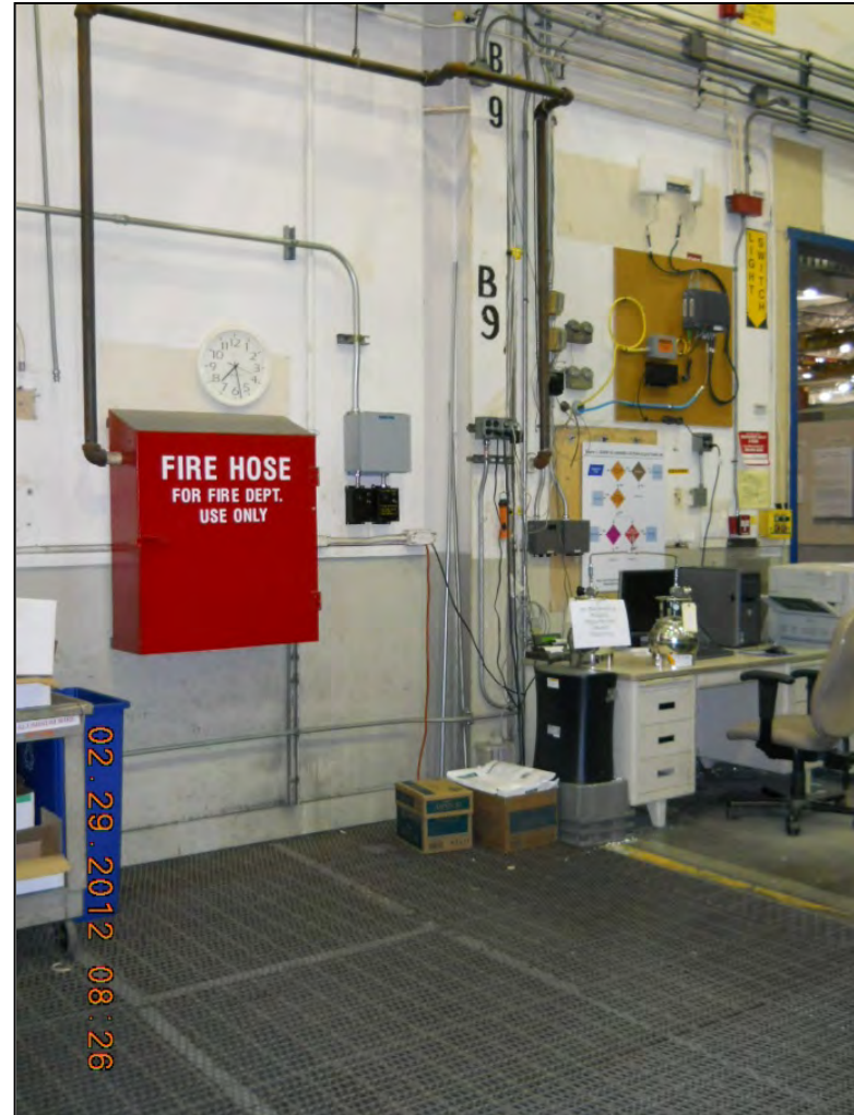
6. Indoor air sample IA04 and duplicate IA99 at Building 17-07 located adjacent to SWMU S-13.
