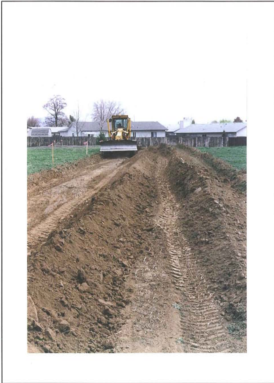
Figure 3: Road grader test plot after cutting to 18 inches.
