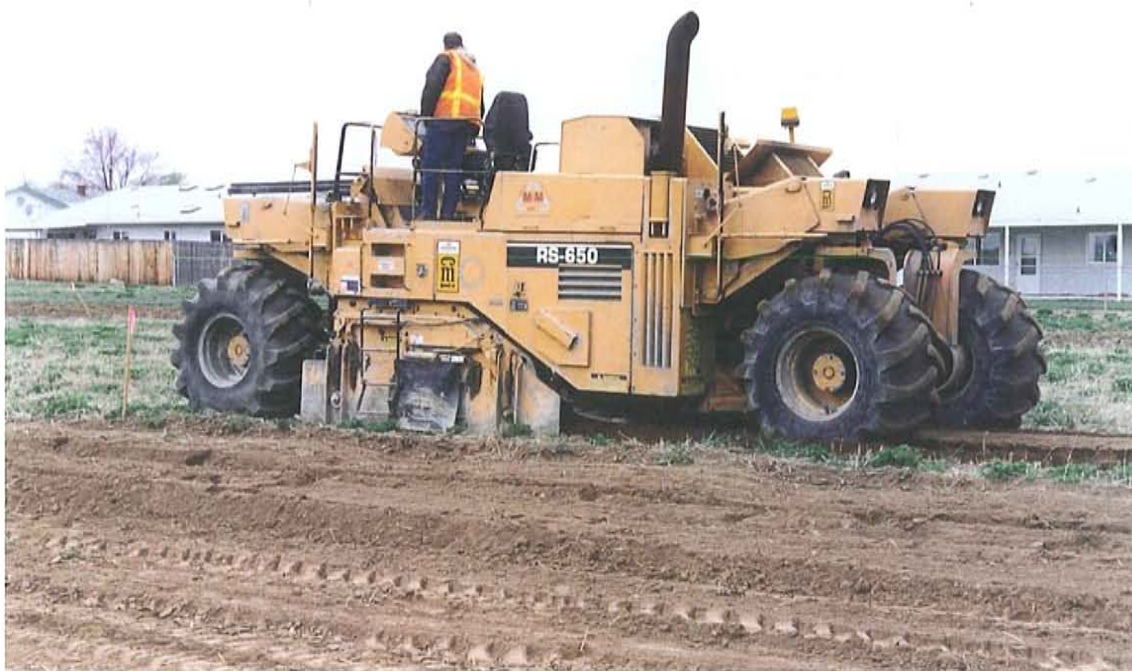
Figure 5: Road reclaimer at N - S test plot.
