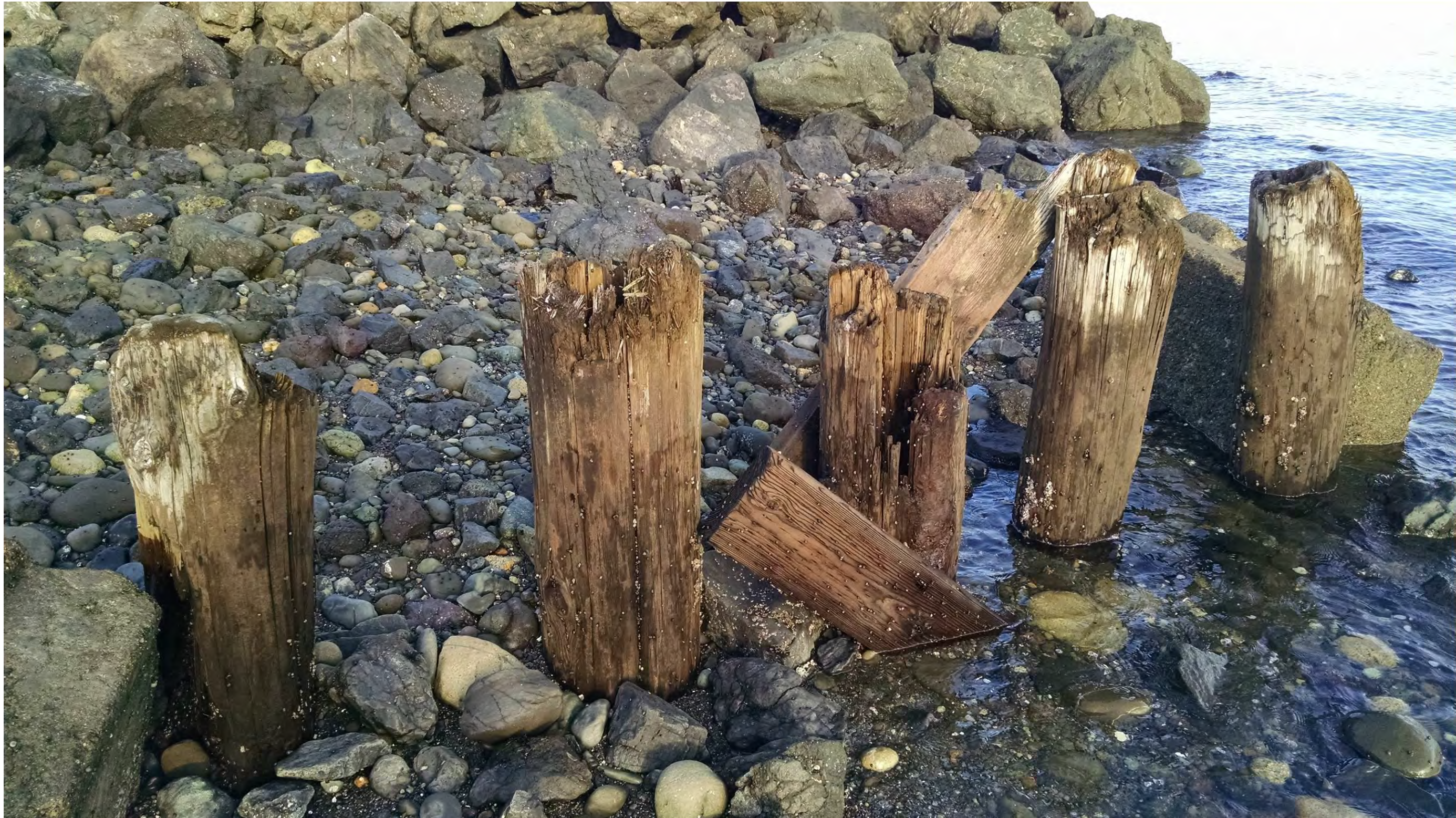
Photo D-5 – Trestle piles at Valley Creek estuary looking northwest.
