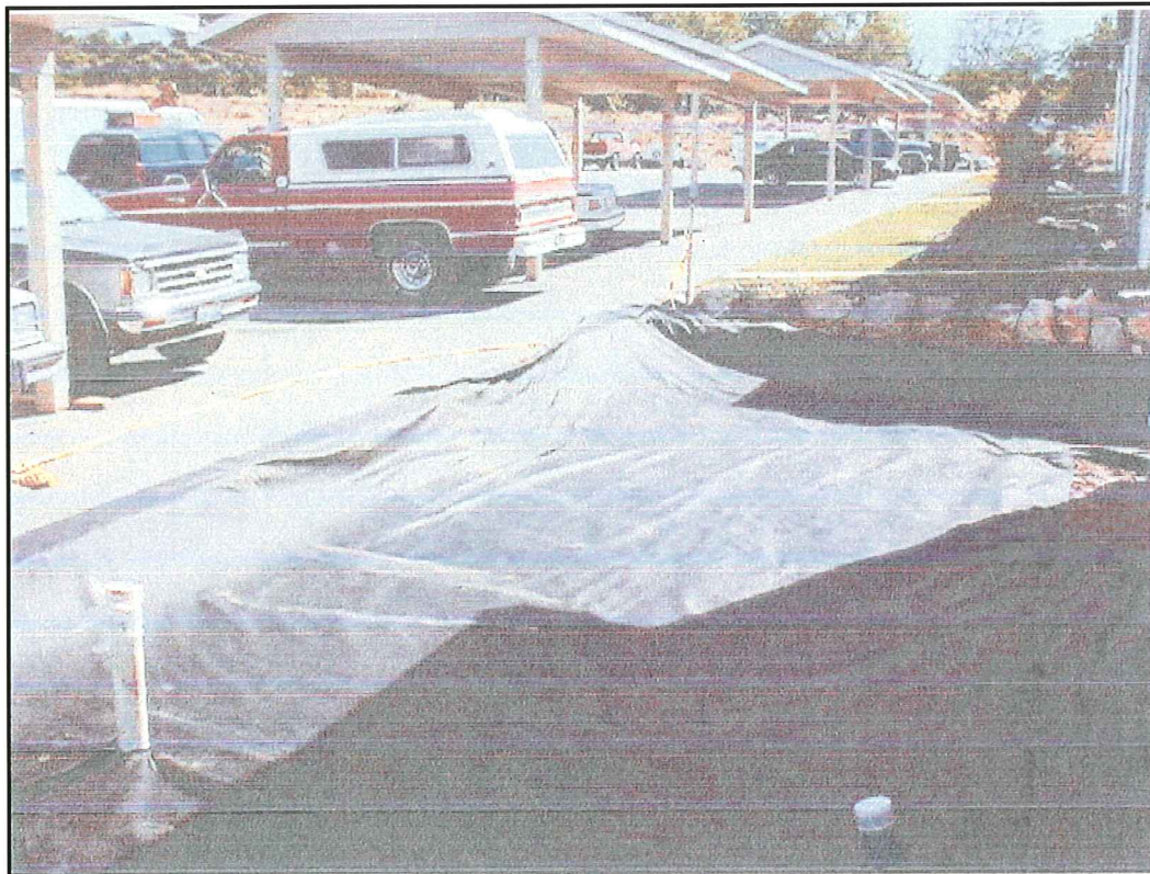
Photo 6: Geotextile along northern perimeter.
