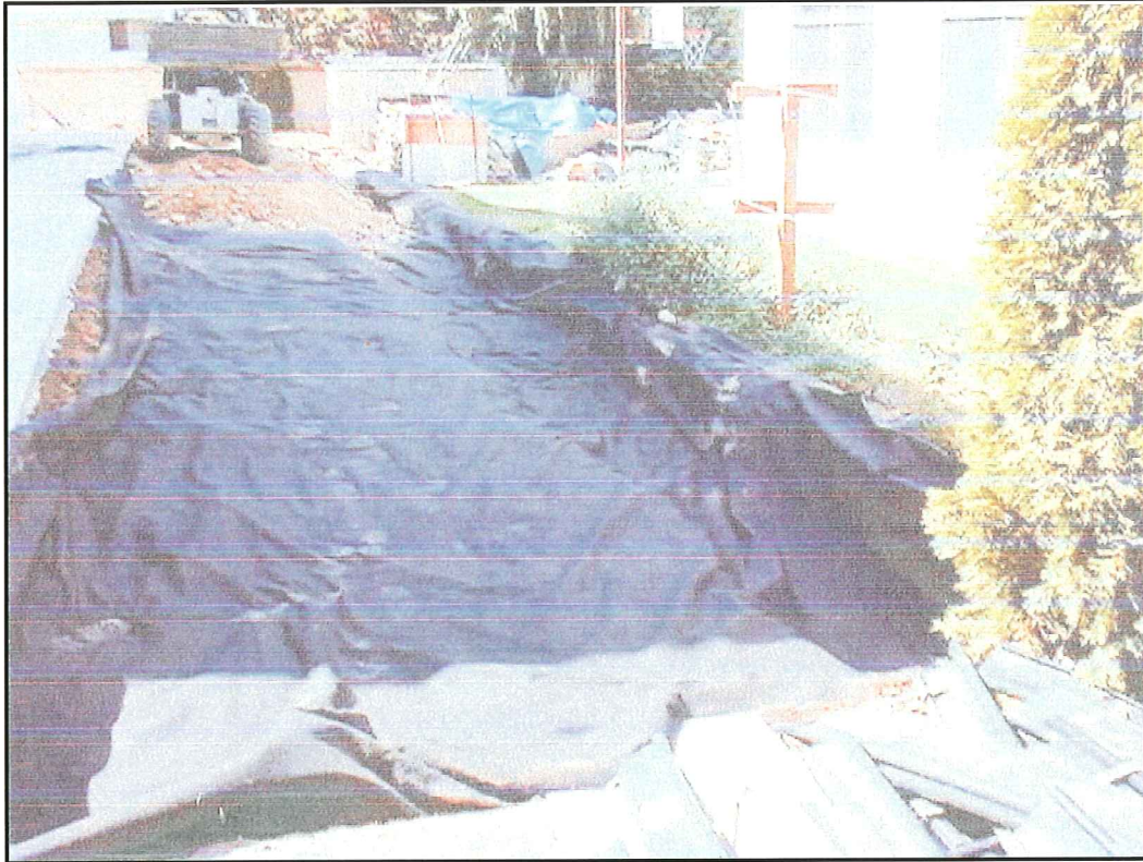
Photo 5: Geotextile along western perimeter.
