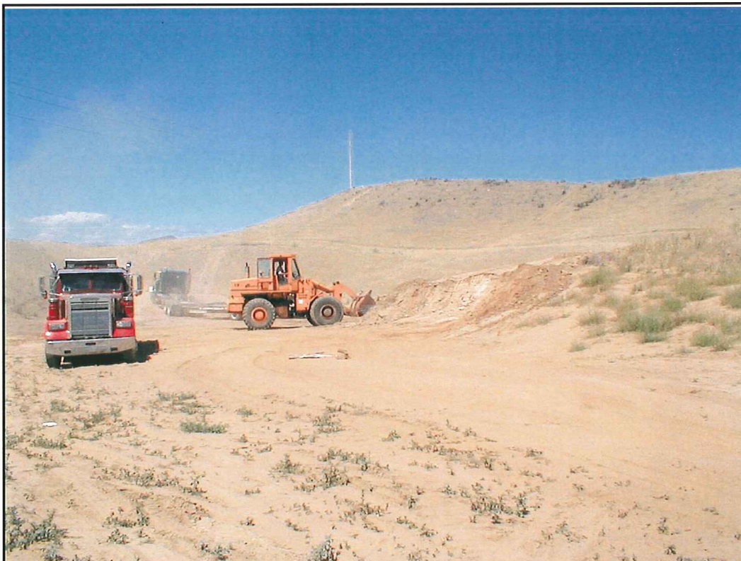
Photo 10: Loading clean topsoil from source on Blue Grade Road.
