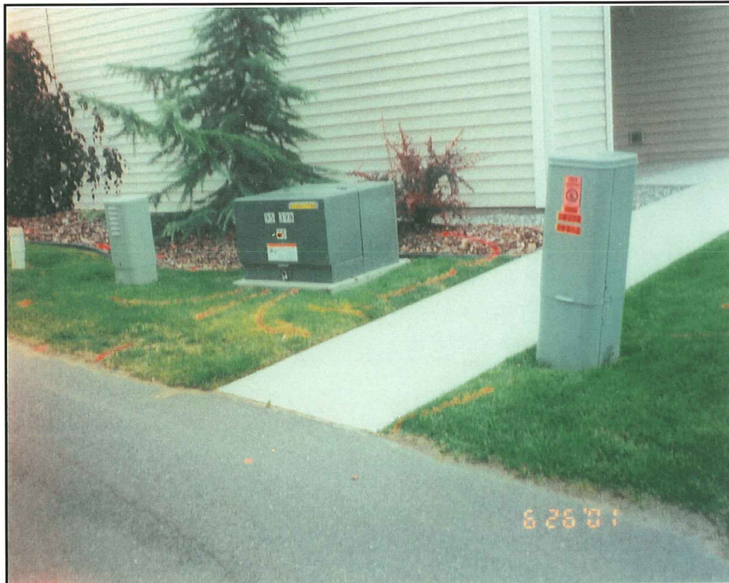
Photo 2: View of transformer/telephone pedestal before excavation activities.
