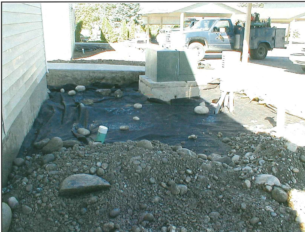
Photo 8: West-facing view of transformer/telephone pedestal during placement of gravel fill.
