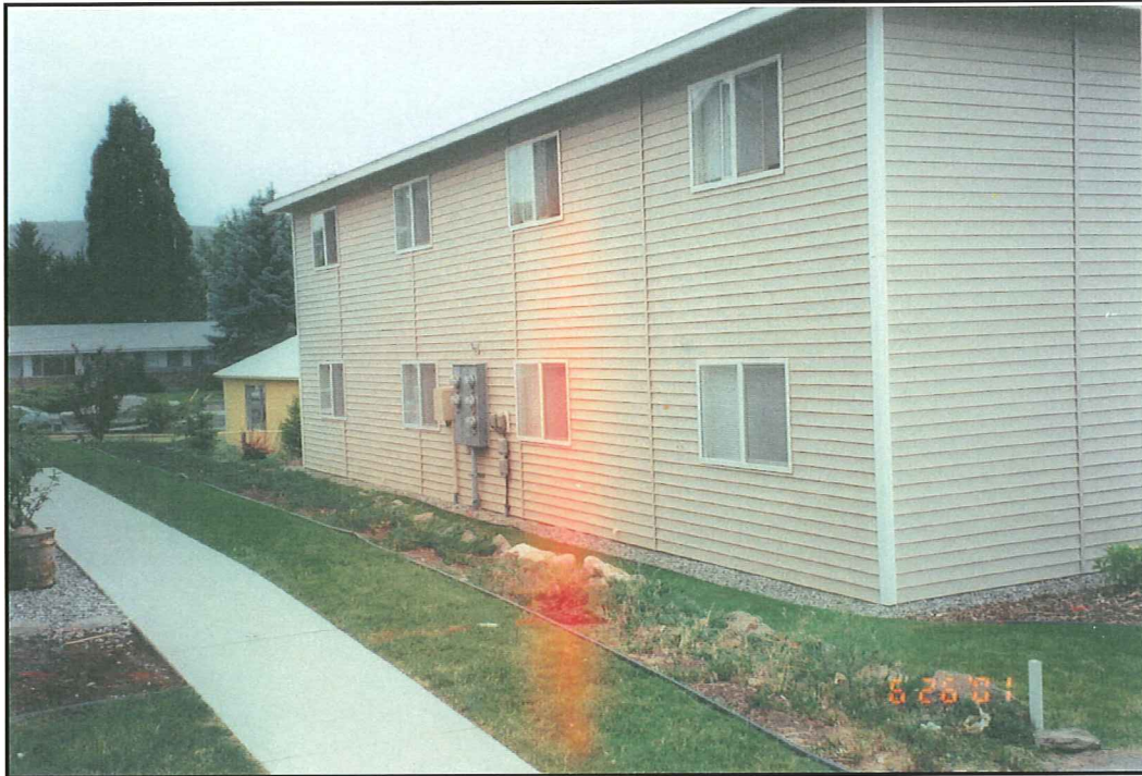
Photo 1: South-facing view between the two structures, 581 and 583, before excavation activities.
