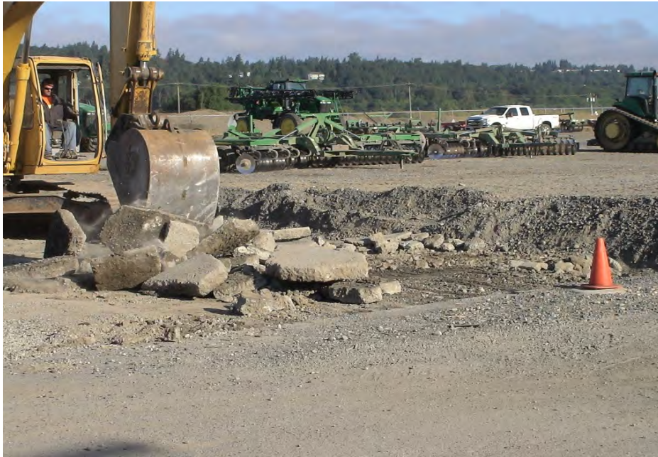
Removal of concrete pad discovered in April 2014
