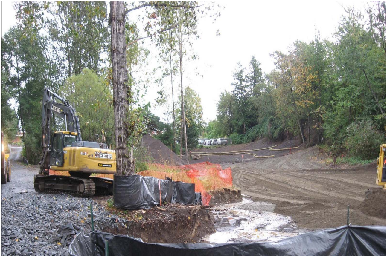
Excavation being backfilled and graded at Eldridge Municipal Landfill site (September 2011).
