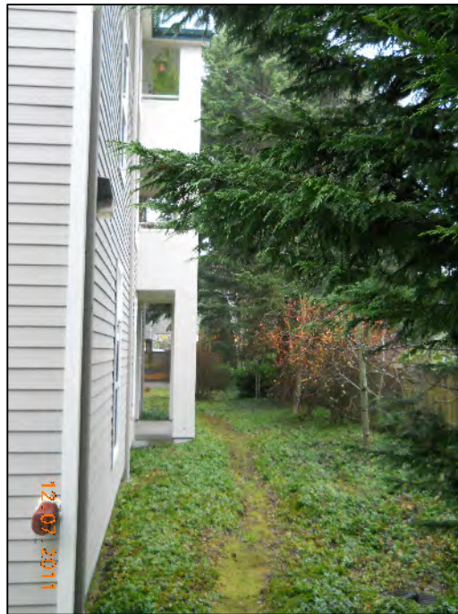
Photograph 6: Looking north along the east side of the building.
