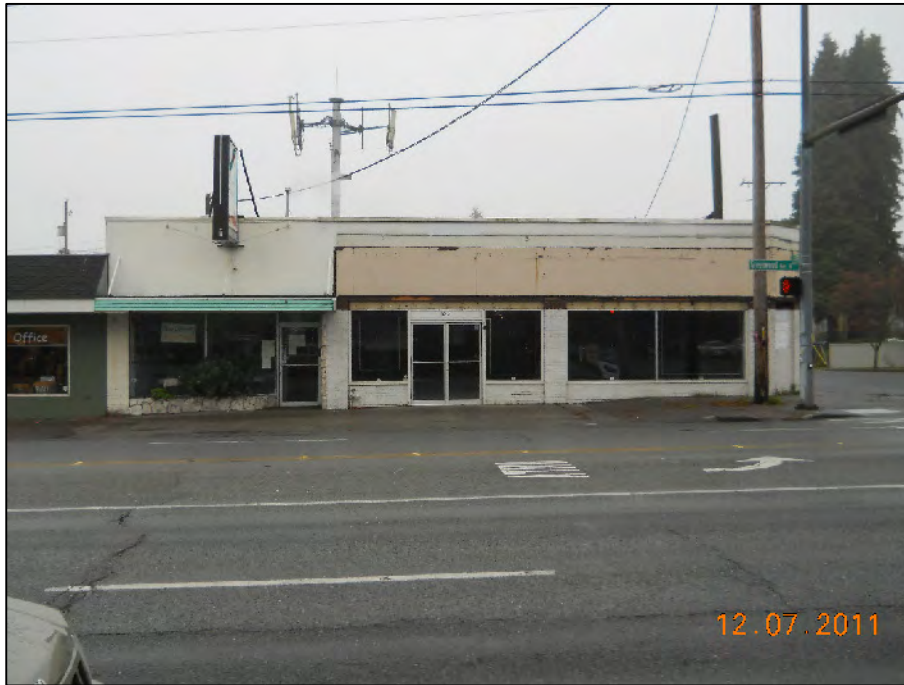
Photograph 27: Looking west at 12427 and 12431 Greenwood Avenue North, a Chinese restaurant and vacant tenant space.
