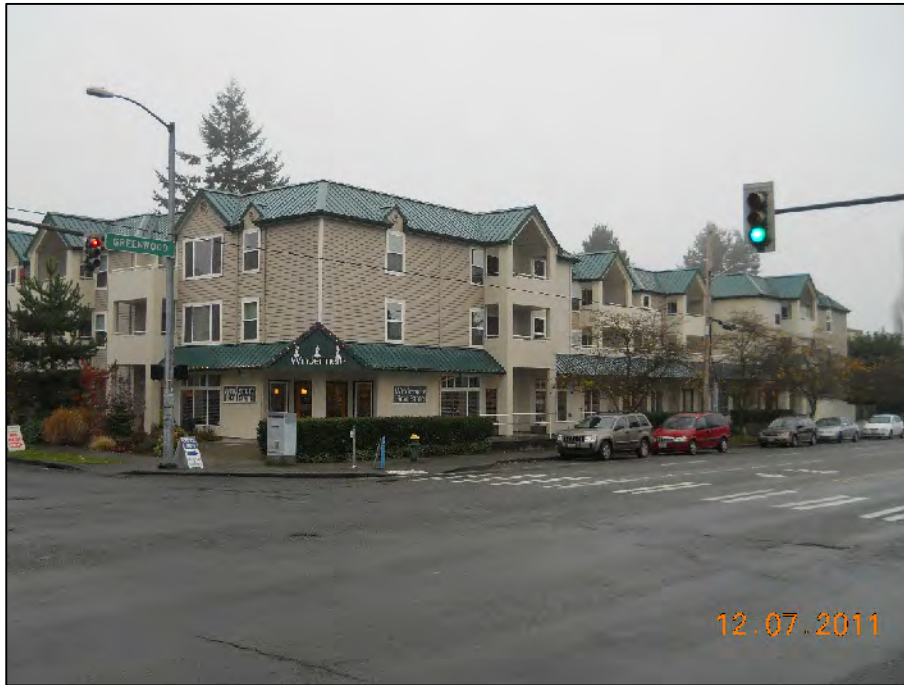
Photograph 1: Looking southeast at the west side of the Site.
