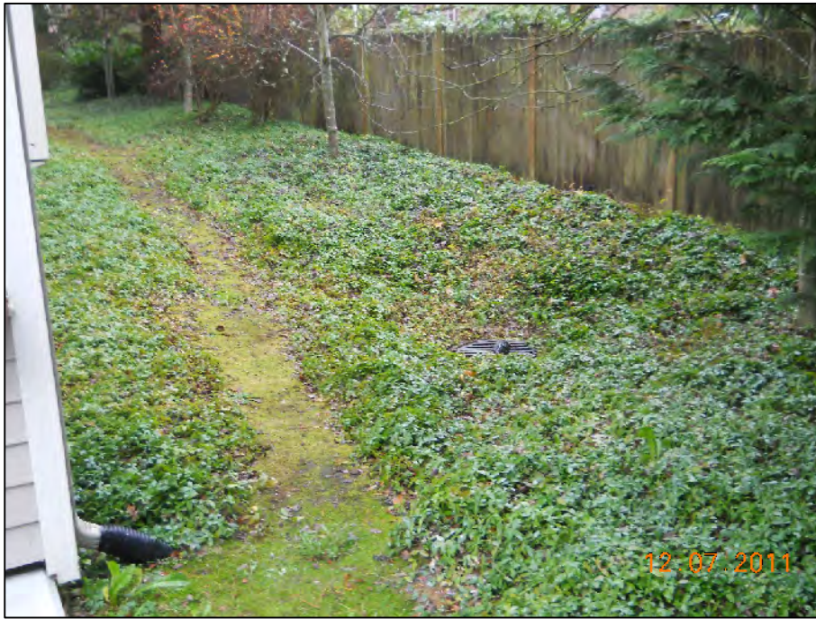
Photograph 7: Ground cover on east side of the building. Note stormwater catch basin that is also fed by roof drains.
