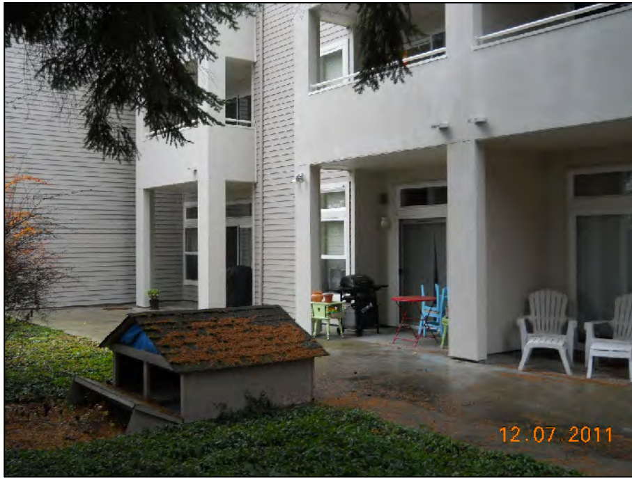
Photograph 9: Looking west at the east side of the building.
