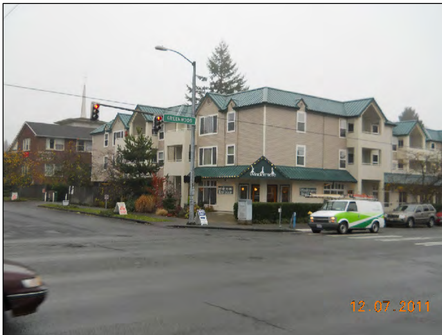
Photograph 2: Looking southeast at the Site. Greenwood Avenue North is in the foreground.
