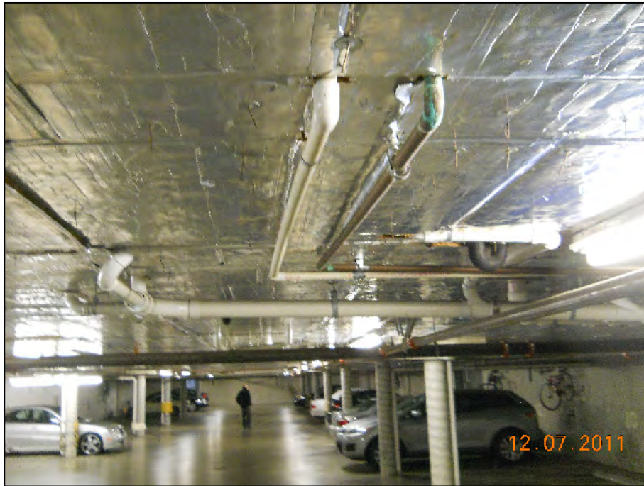
Photograph 11: Looking north in the parking garage.
