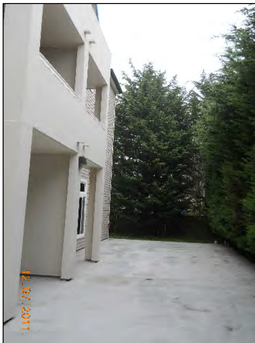
Photograph 4: Looking east along the south side of the building.
