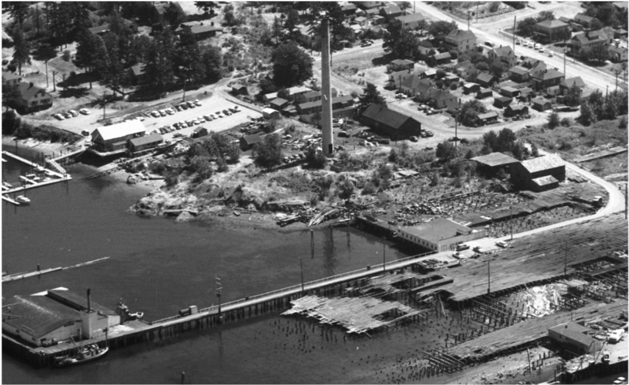
Photo 4: Circa 1959 aerial photograph of the Robinson Marina and surrounding area (Courtesy of Port of Anacortes).
