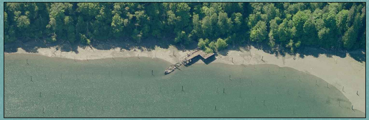
PHOTO 10: FORMER LOG TRANSFER FACILITY (FROM BING MAPS IMAGERY)
