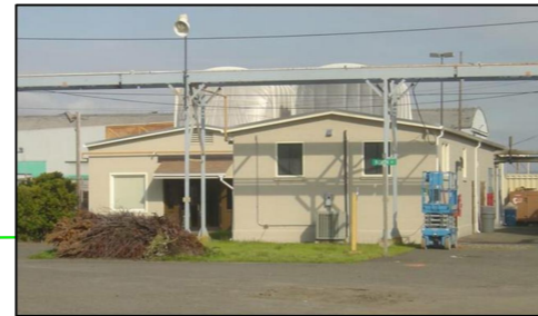
EXTERIOR VIEW - WEST SIDE
