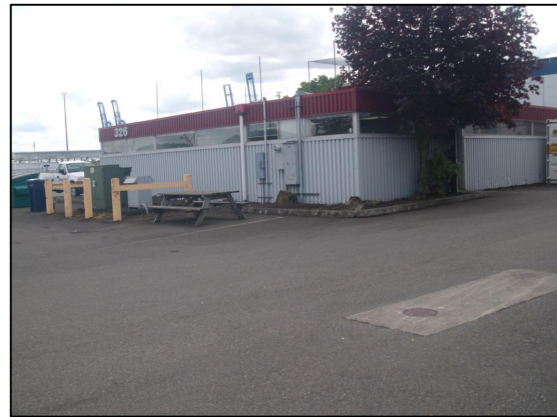
EXTERIOR VIEW - NORTHEAST CORNER
