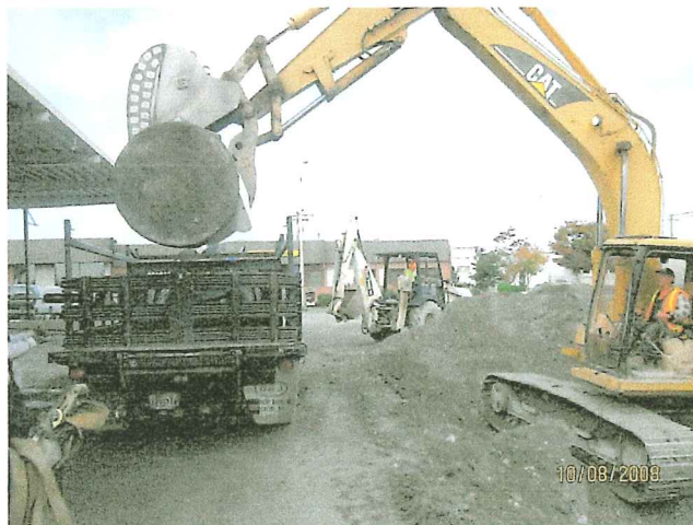
Photo of tank being loaded for transport
