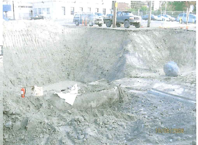
Photo of UST prior to removal
