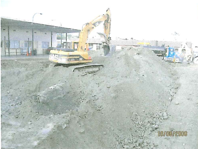
Photo of UST Location (prior to removal)
