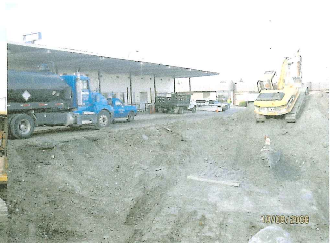
Photo of remedial excavation
