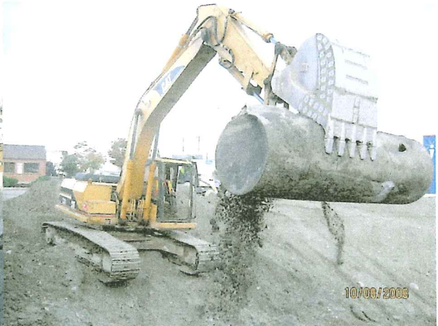
Photo of tank during removal
