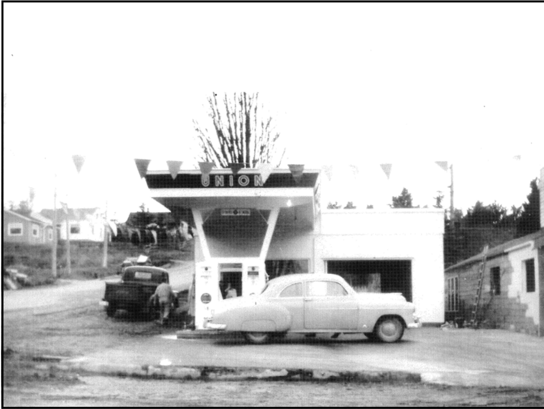
Photograph 1. Photo date unknown. Photo provider states that the gas station was a Union gas station constructed in 1951/1952 next to the auto body shop that was constructed in 1950.
