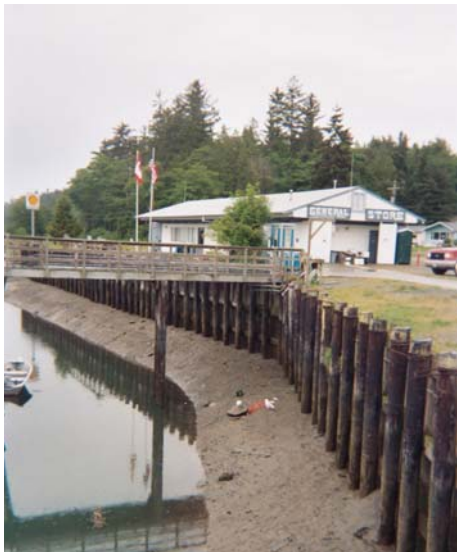
View of Cornet Bay Marina Site Looking North Toward Store
