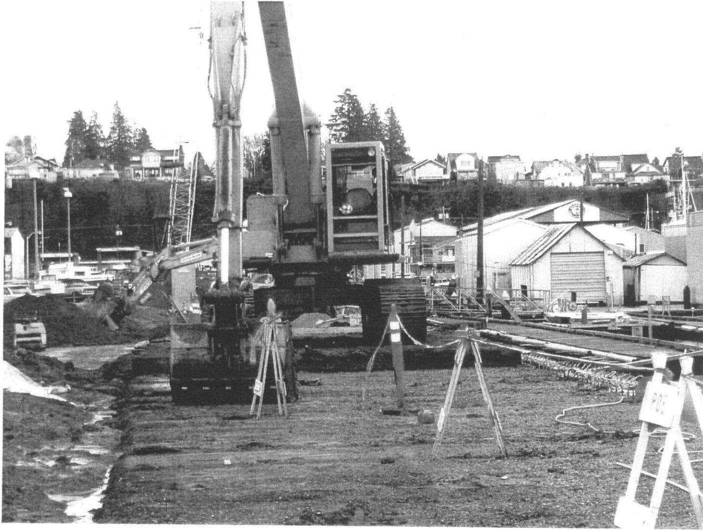
Figure 6. Equipment on Timber Raft.
