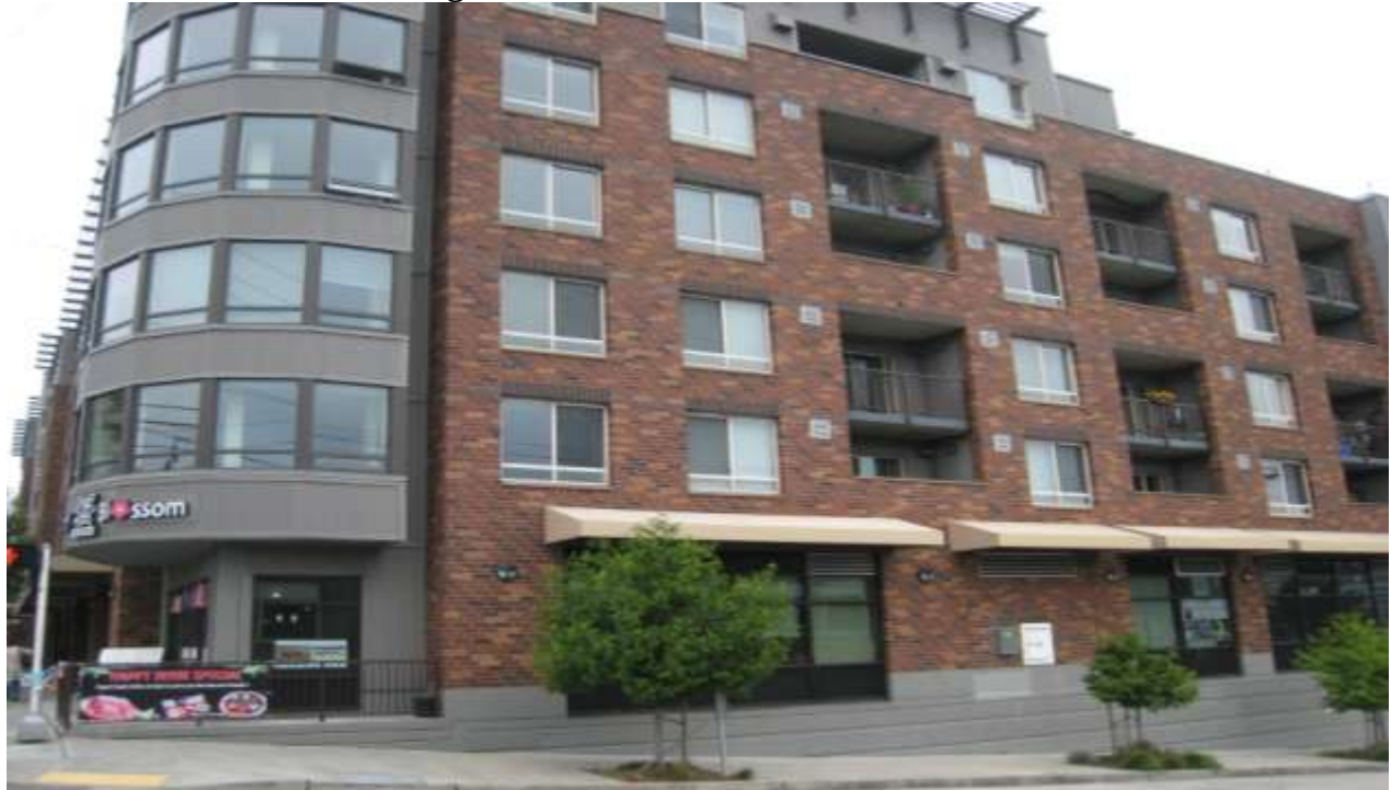
Photo 2: South side of the bldg. - from the south across Aloha
