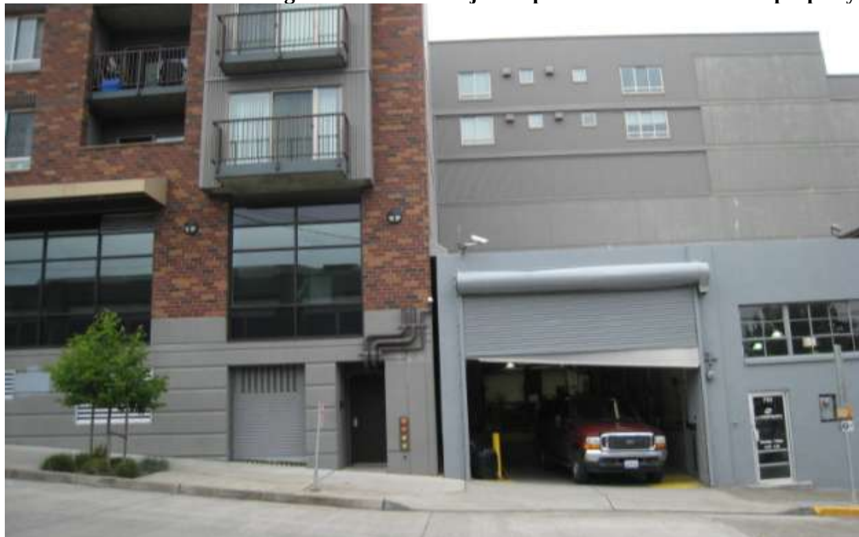
Photo 4: South Side of the bldg. where it meets adjacent parcel – cont. extends off-property
