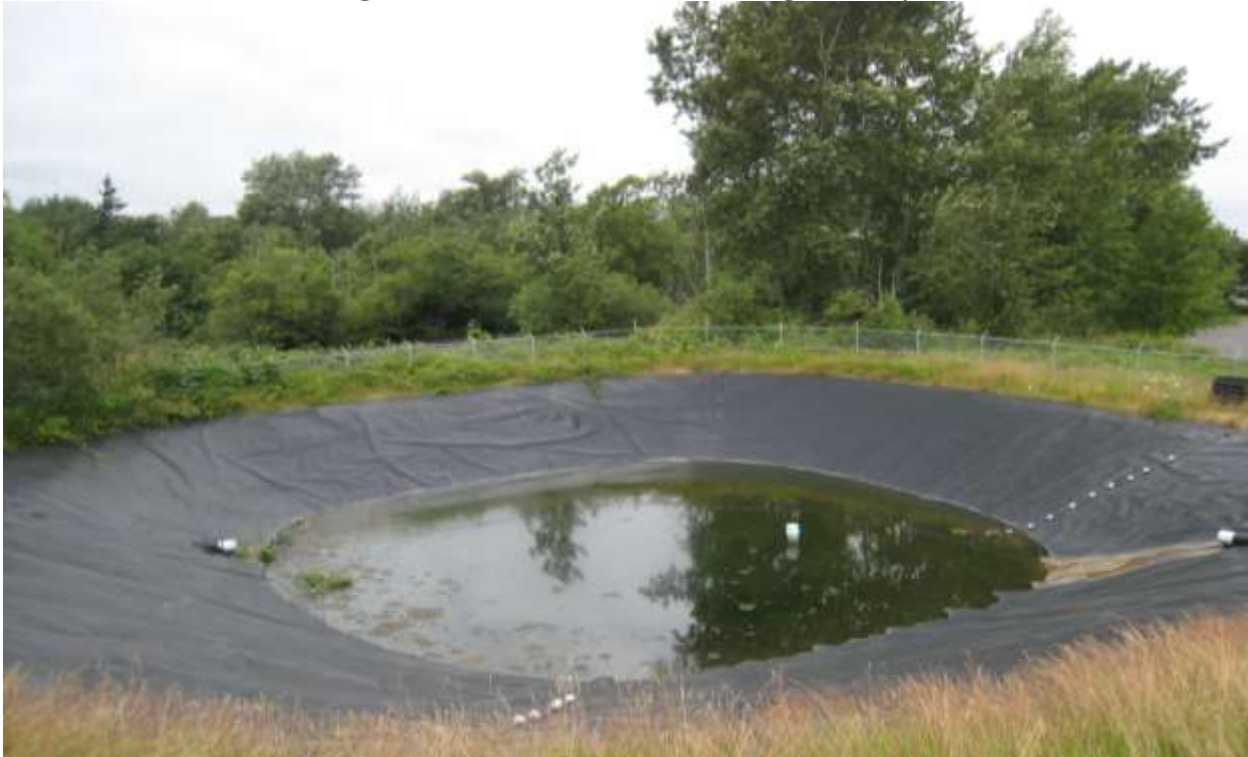
Photo 4: Lined leachate lagoon collects water from underground system
