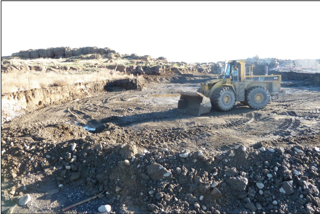
Photo 9: Bedrock scraping western part of excavation (looking east)
