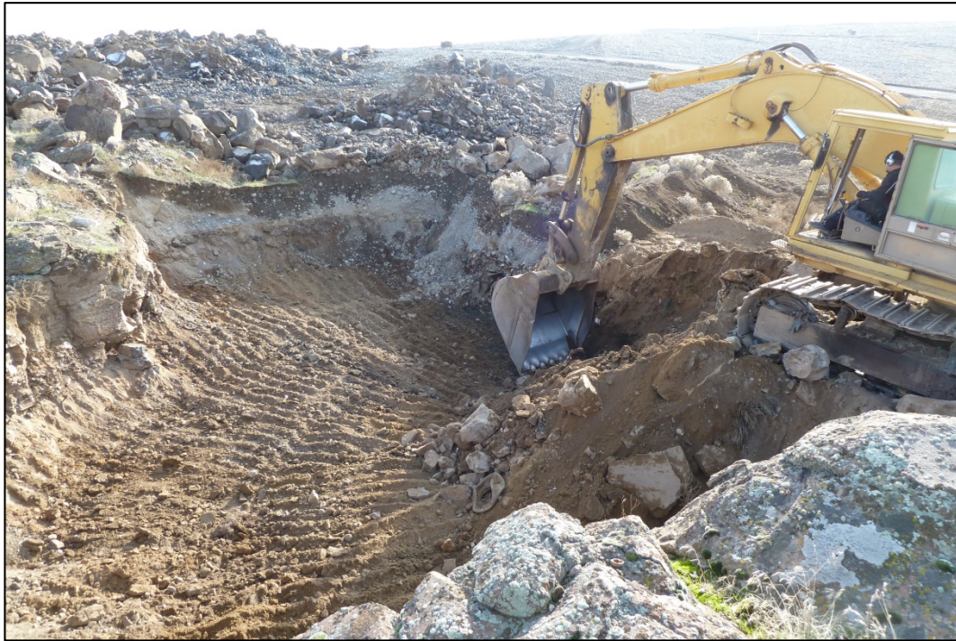
Photo 1: Soil removal method using track hoe (looking south)
