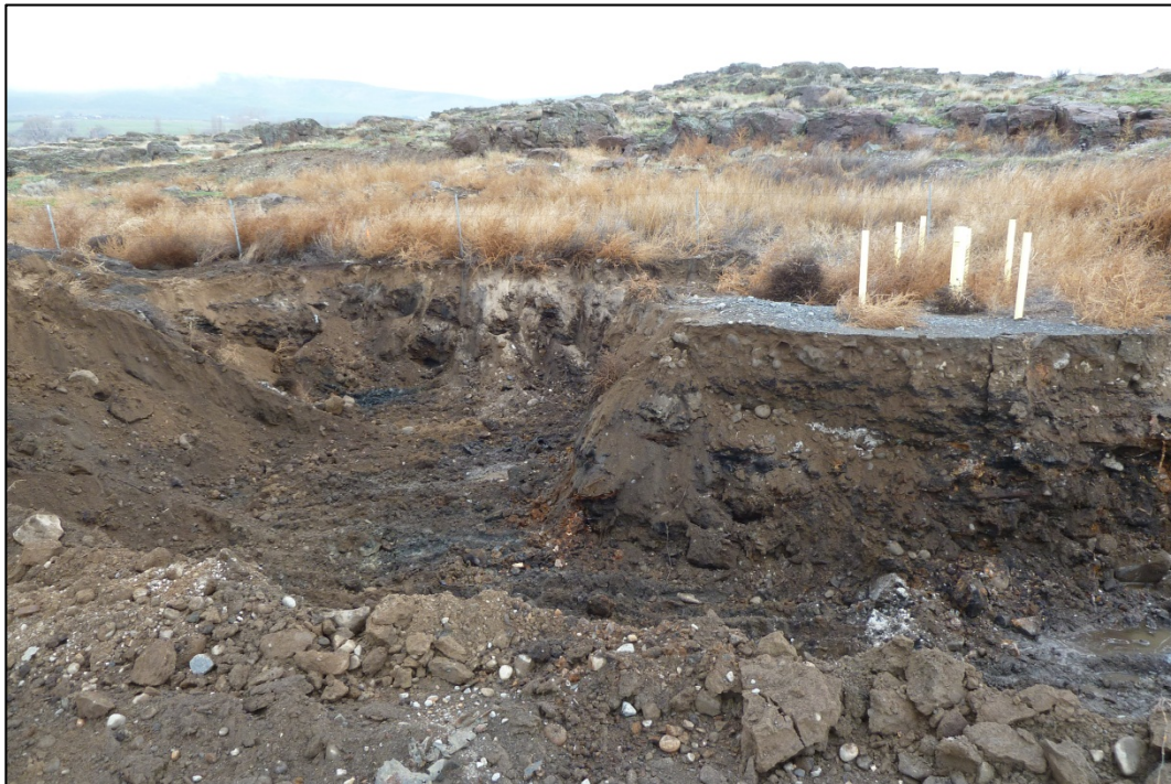
Photo 6: Soils left in place around MW-41a and MW-40p2 (looking north)
