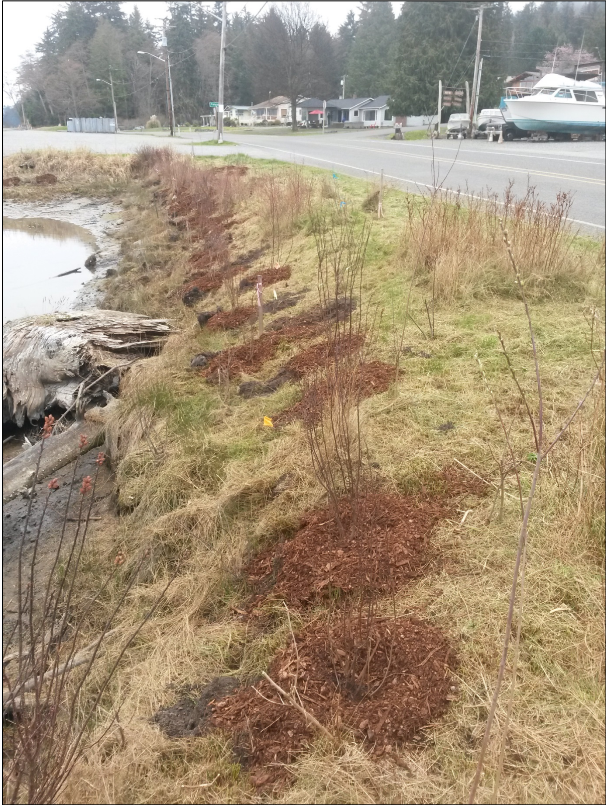
Photograph 1. Sweet gale installed along southeast portion of the wetland enhancement area
