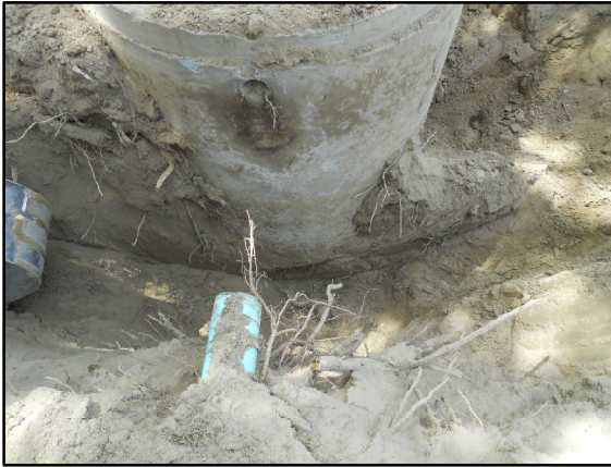
C. New septic system : East Concrete Tank
