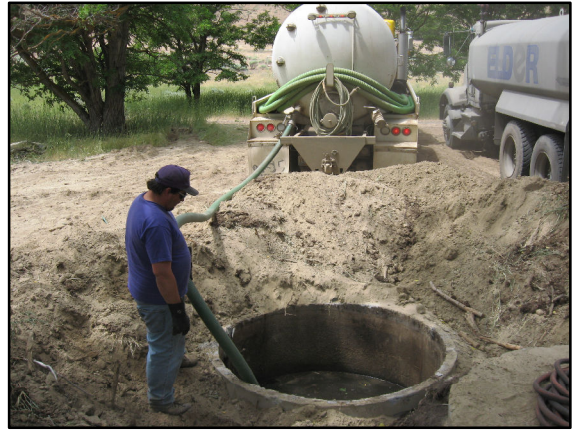
D. West concrete tank
