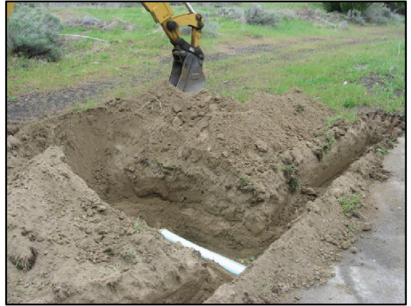
B. New septic underneath west side of office building
