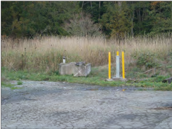
P8 VIEW OF THE NORTHEAST CORNER OF FENCED AREA AND MONITORING WELL GEI-MW6 AND MW3; LOOKING NORTHEAST (NOVEMBER 2009)
