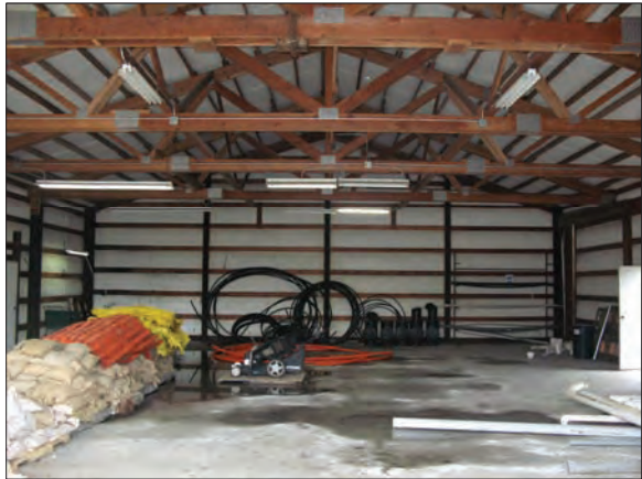
P5 INSIDE VIEW OF THE HANGAR BUILDING (CONCRETE PORTION) CONTENTS INSIDE OF BUILDING TO BE REMOVED PRIOR TO CONSTRUCTION; LOOKING SOUTH (MARCH 2011)
