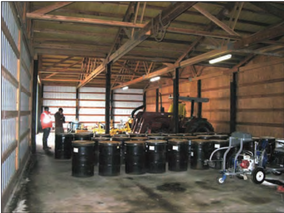
P6 INSIDE VIEW OF THE HANGAR BUILDING (ASPHALT PORTION) CONTENTS INSIDE OF BUILDING TO BE REMOVED PRIOR TO CONSTRUCTION; LOOKING EAST (MARCH 2011)
