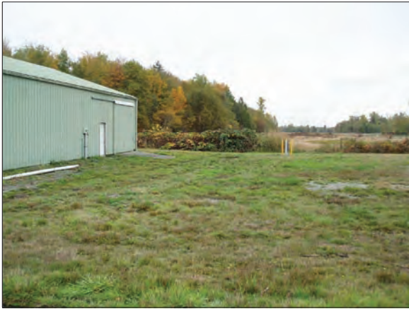
P4 VIEW OF WESTERN WALL OF HANGAR BUILDING AND SURROUNDING AREAS; LOOKING SOUTHEAST (OCTOBER 2009)
