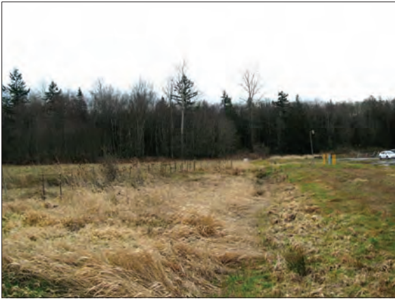
P2 VIEW OF DRAINAGE CHANNEL (NORTH OF ASPHALT DRIVEWAY); LOOKING EAST (MARCH 2011)
