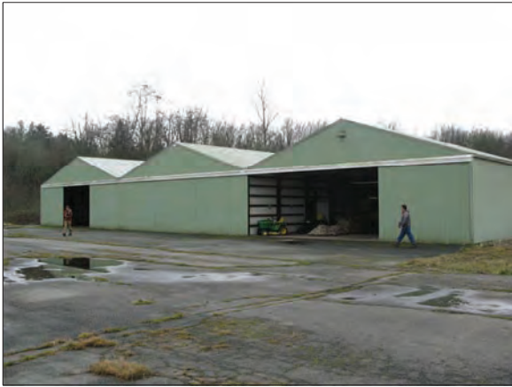
P3 FRONT VIEW OF HANGAR BUILDING AND ASPHALT DRIVEWAY; LOOKING SOUTHEAST (MARCH 2011)
