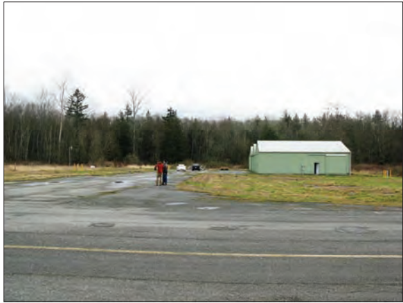
P1 VIEW OF TAXIWAY F, ASPHALT DRIVEWAY AND SIDE VIEW OF HANGAR BUILDING; LOOKING EAST (MARCH 2011)
