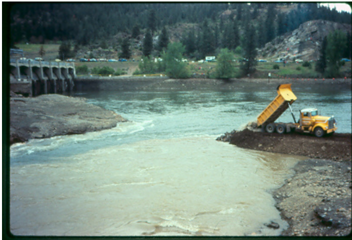
Photo 4. Repairs at Mouth of Powerhouse Intake Channel
