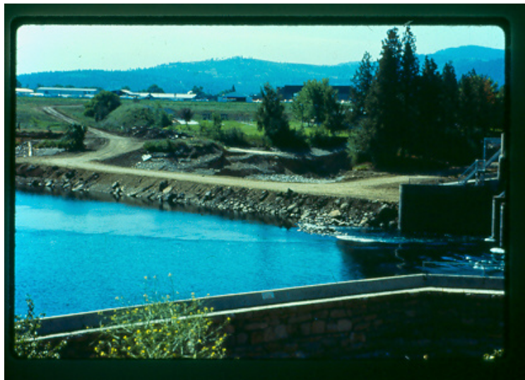
Photo 6. Repairs South of Dam Face from Upstream
