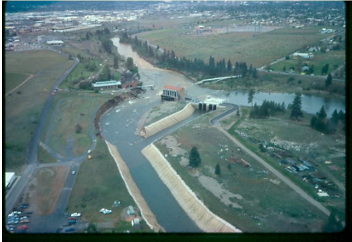
Photo 1. Aerial View of Powerhouse Intake Channel and Powerhouse
