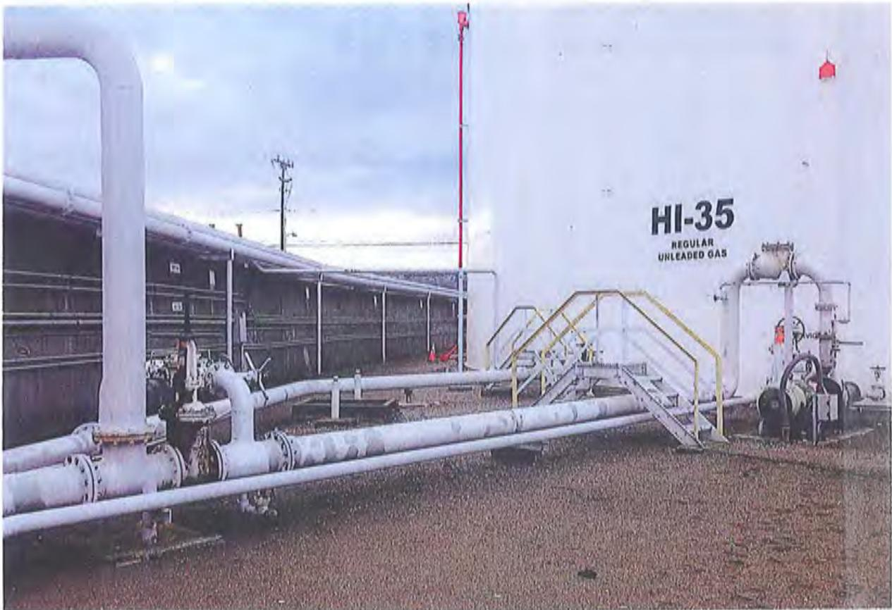
Photo 4. KMLT Above ground petroleum Storage Tank No 35 at E Yard with supply piping and valves.
