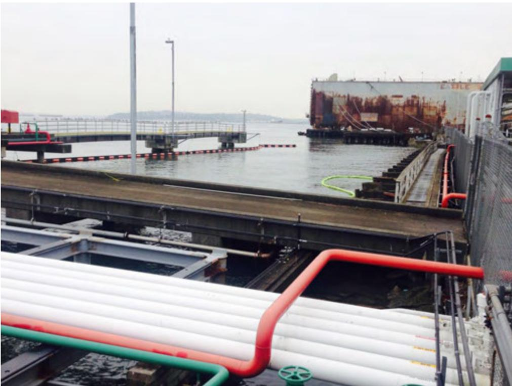
Photo 2. BP Terminal seawall parallel to loading rack on right, green boom to capture any sheen or floating product on West Waterway is a safety measure. Foreground is piping for on-loading and off-loading petroleum from barges or ships at West Waterway. Left is barge and ship dock with Elliott Bay is in background.
