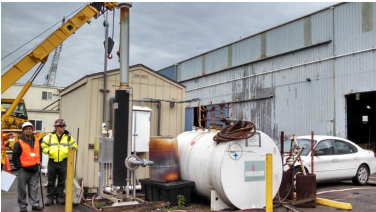
Photo 18. West LNAPL Shed LNAPL tank and catalytic oxidizer
