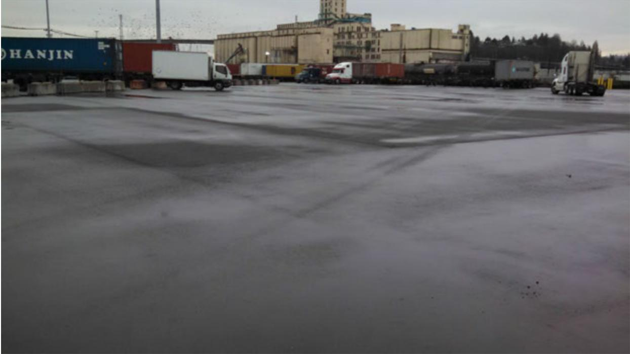
Photo 8. Minimal water ponding after regrading and capping
