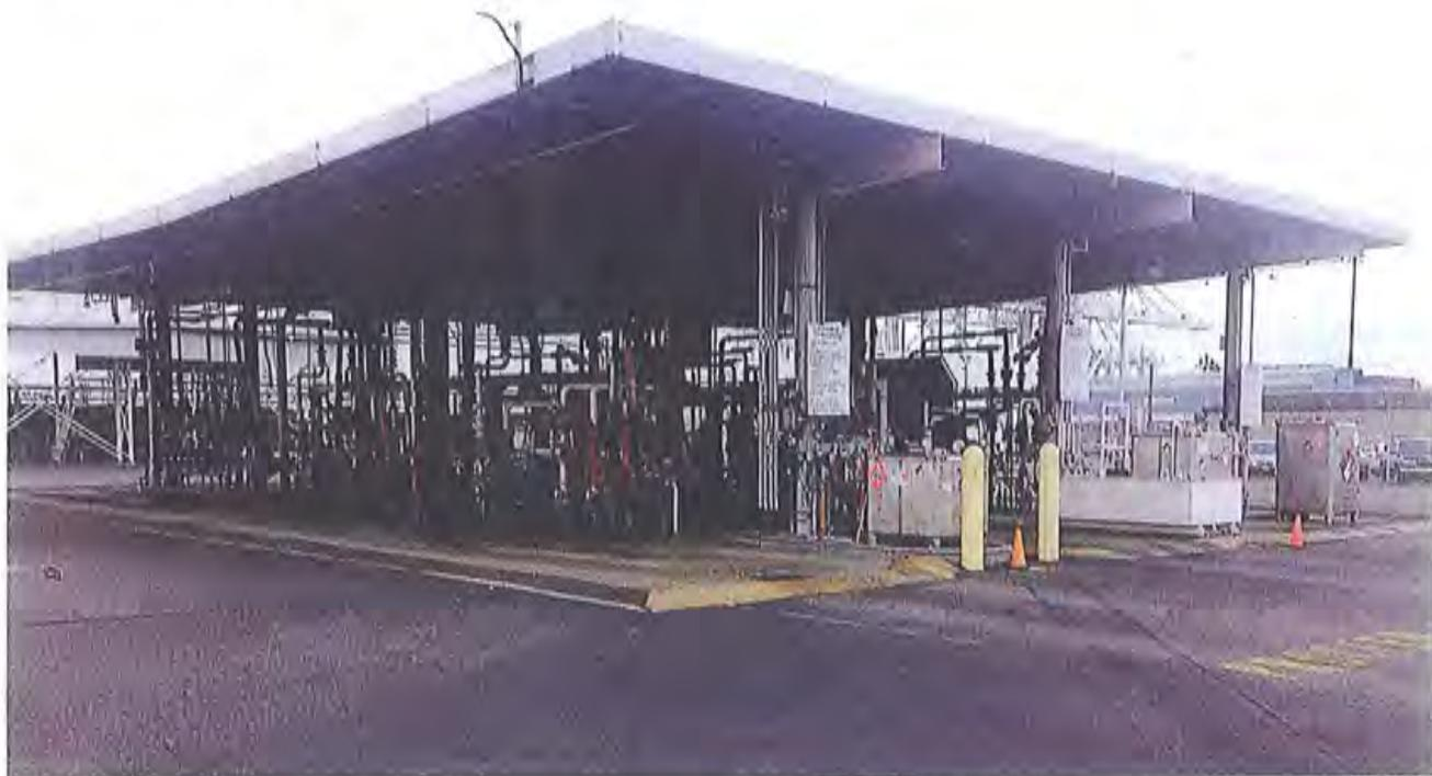
Photo 1. KMLT illustrating a petroleum fuels loading rack.
