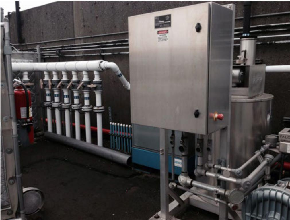
Photo7. BP Terminal Soil Vapor Extraction Remediation System equipment is shown with pumping station, vapor removal and stripping system and six individual well piping with control valves. This system is removing petroleum vapors from soil and groundwater for subsurface cleanup action.
