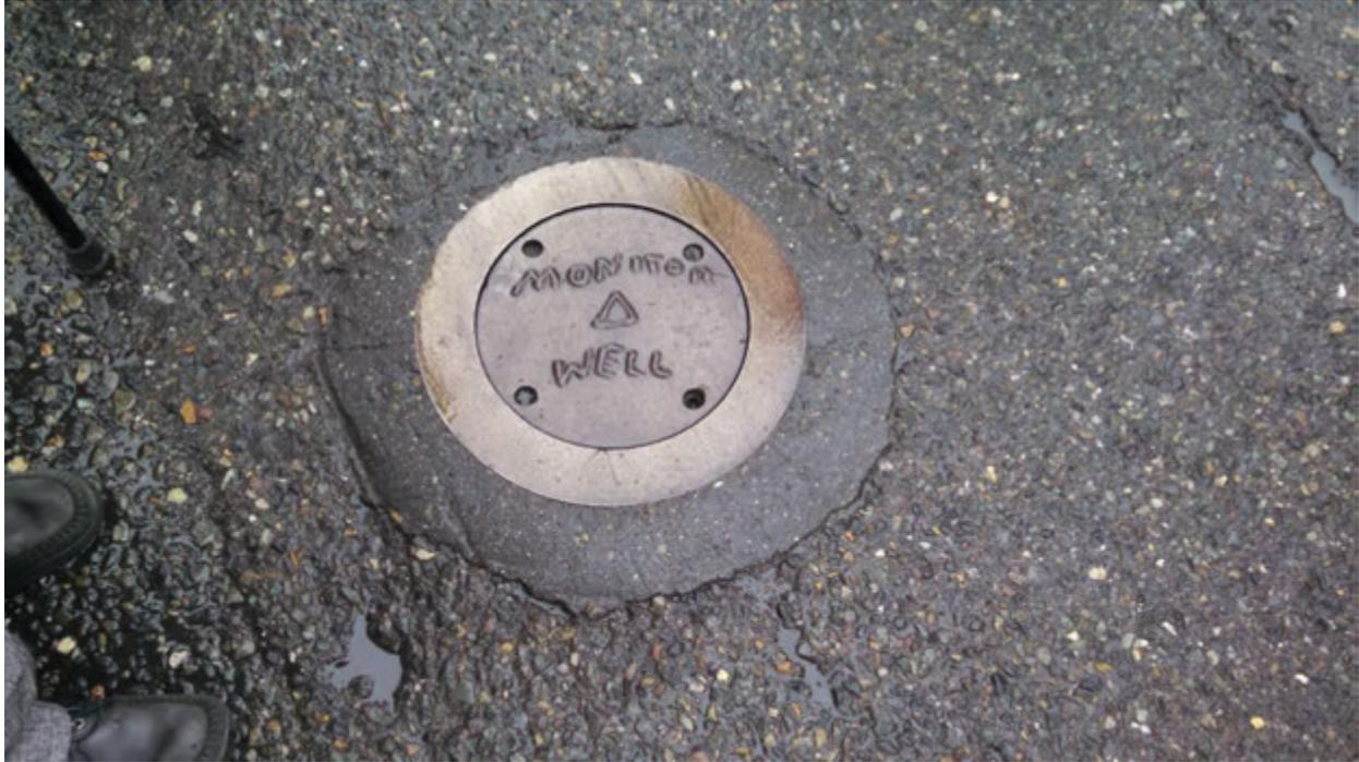
Photo 5. Monitoring well HI-3 (bolts missing)
