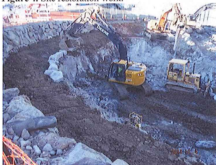
Figure 4. Site restoration work.
