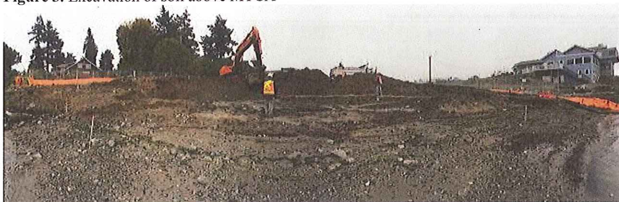
Figure 3. Excavation of soil above MTCA
