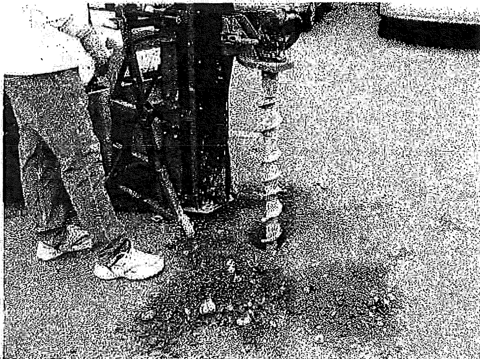
Exploration of Boring B2 at the parking lot
