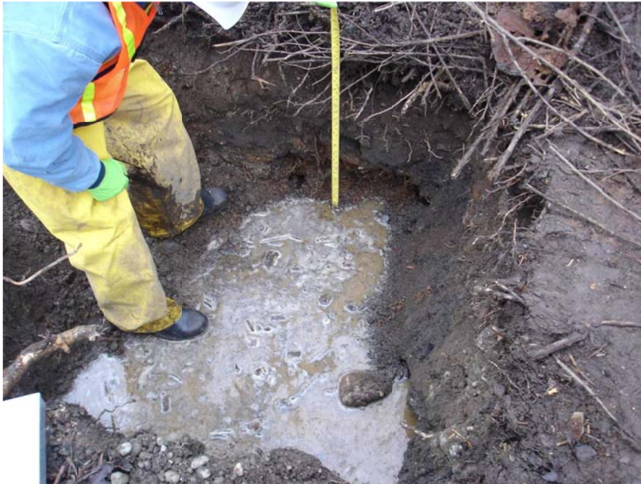
TP-22 West Sidewall
