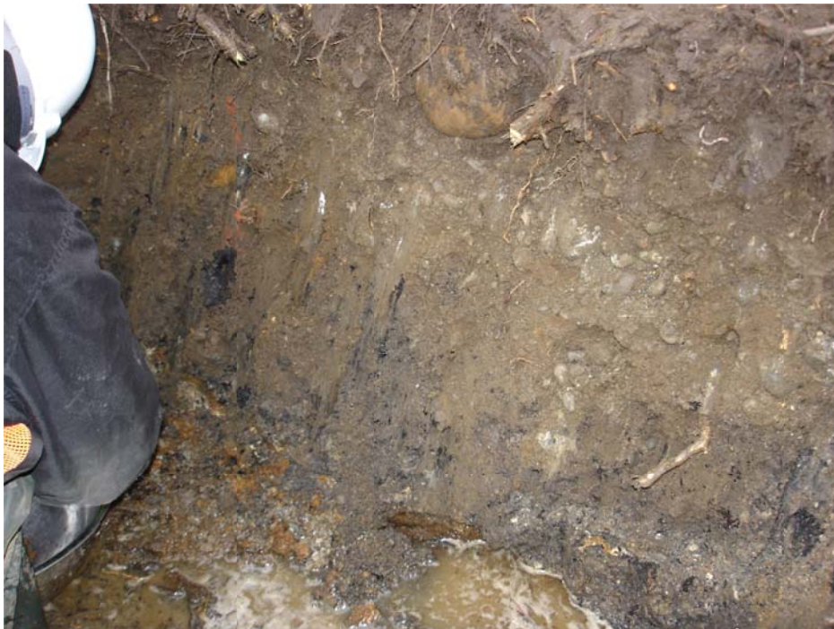
TP-22 South Sidewall
