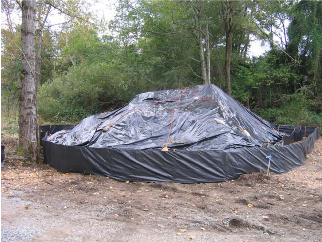
Stockpile covered with surrounding silt fence.
