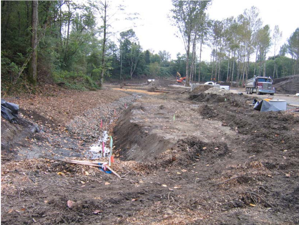
Confirmation sampling locations from western sidewall/slope of BTC/Birchwood Channel.
