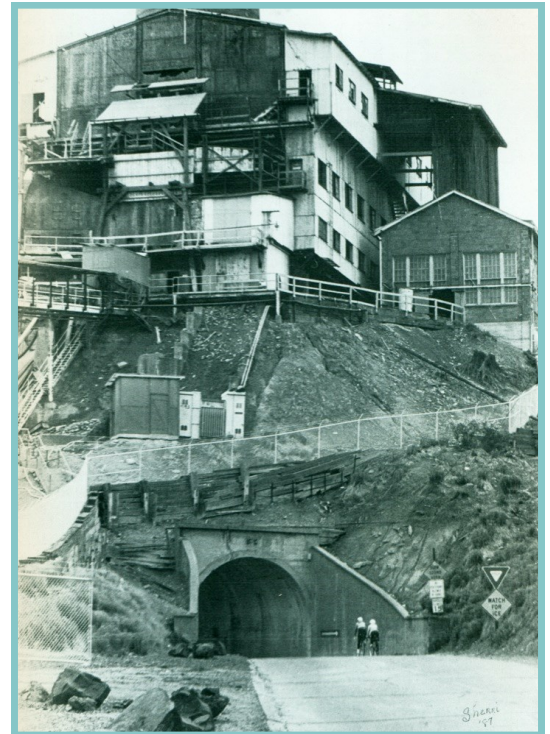
Ruston Tunnel under the former Asarco plant Photo courtesy of Sherri Forch
