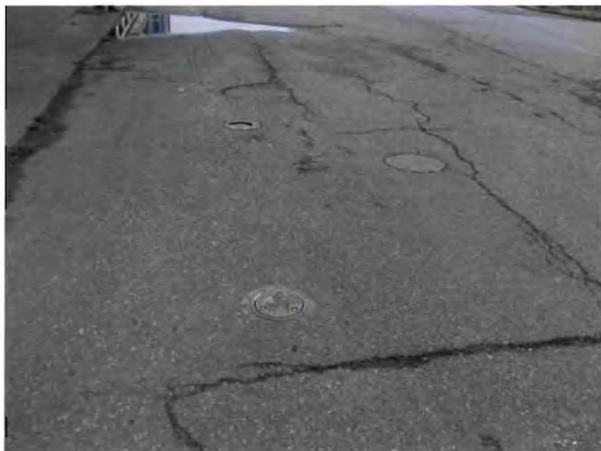
Photo 4 – Active and abandoned monitoring wells along west edge of property in 8 th Avenue.
