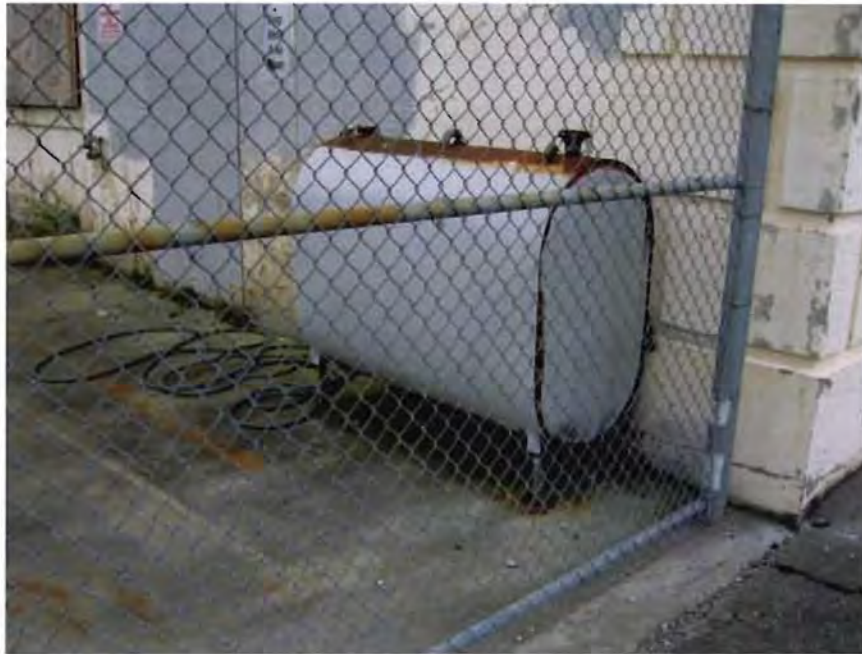
Photo 9 – Aboveground oil storage tank at northwest corner of building.
