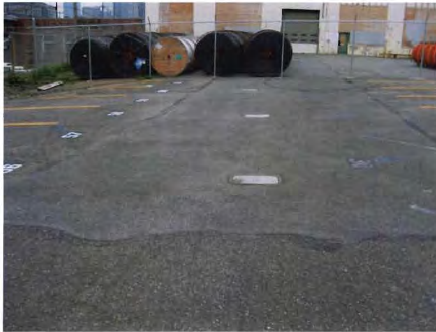
Photo 1 – Possible air sparge well heads in parking lot at north end of property.
