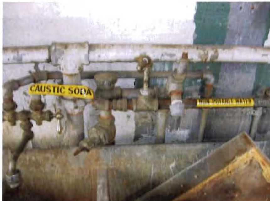
Photo 28 – Closeup of cleaning area in maintenance shop in southern portion of building main floor.
