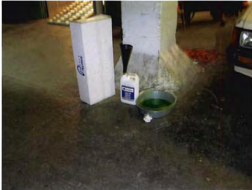
Photo 19 – Coolant usage in central portion of basement.
