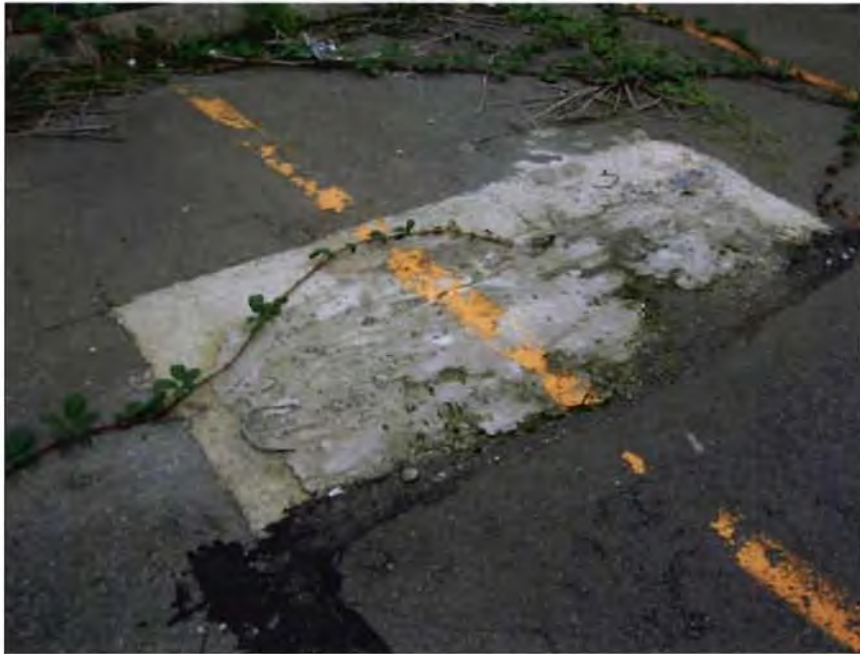
Photo 7 – Possible concrete pad for air sparge and soil vapor extraction equipment.
