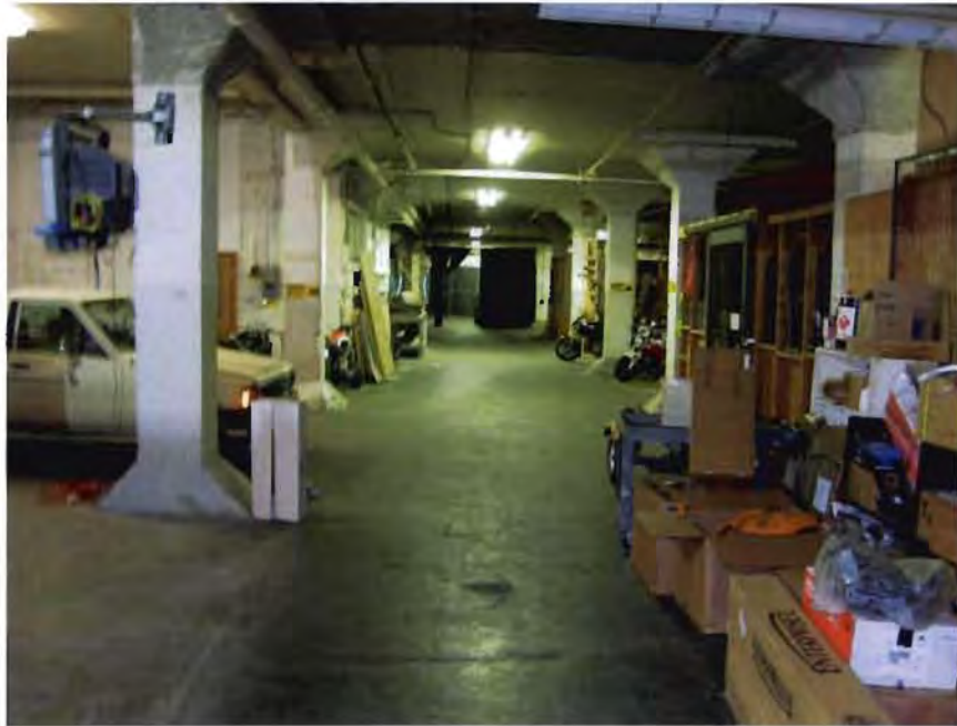
Photo 17 – General view of basement looking south.
