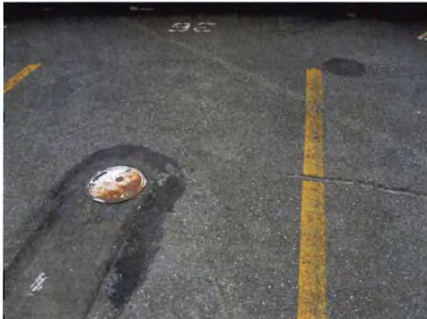
Photo 6 – Possible vapor extraction well head in parking lot at north end of property.
