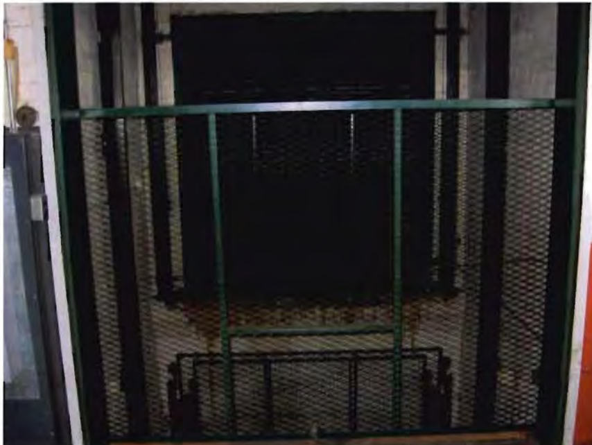
Photo 26 – Utility elevator in central portion of building main floor.
