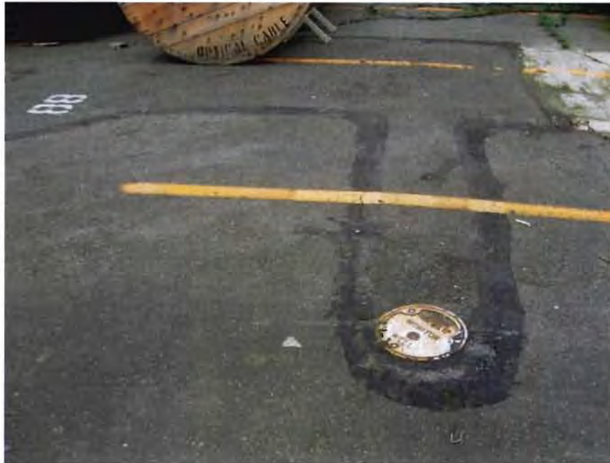
Photo 5 – Possible vapor extraction well head in parking lot at north end of property.
