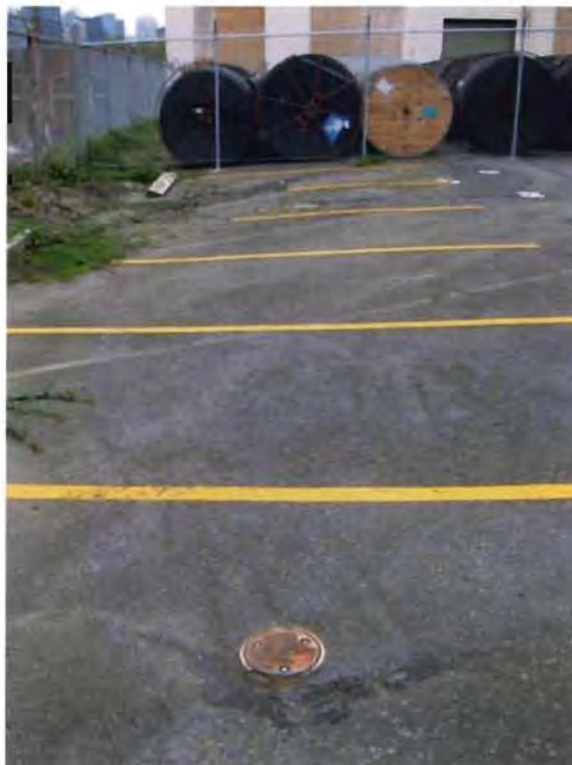
Photo 2 – Possible vapor extraction well head in parking lot at north end of property.
