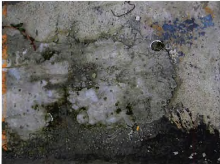
Photo 8 – Closeup of possible concrete pad for air sparge and soil vapor extraction equipment.
