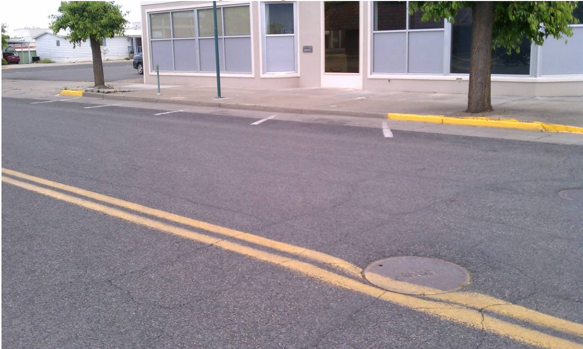
Photo 2: CD-East w/ CNG Building in Background – from the southeast
