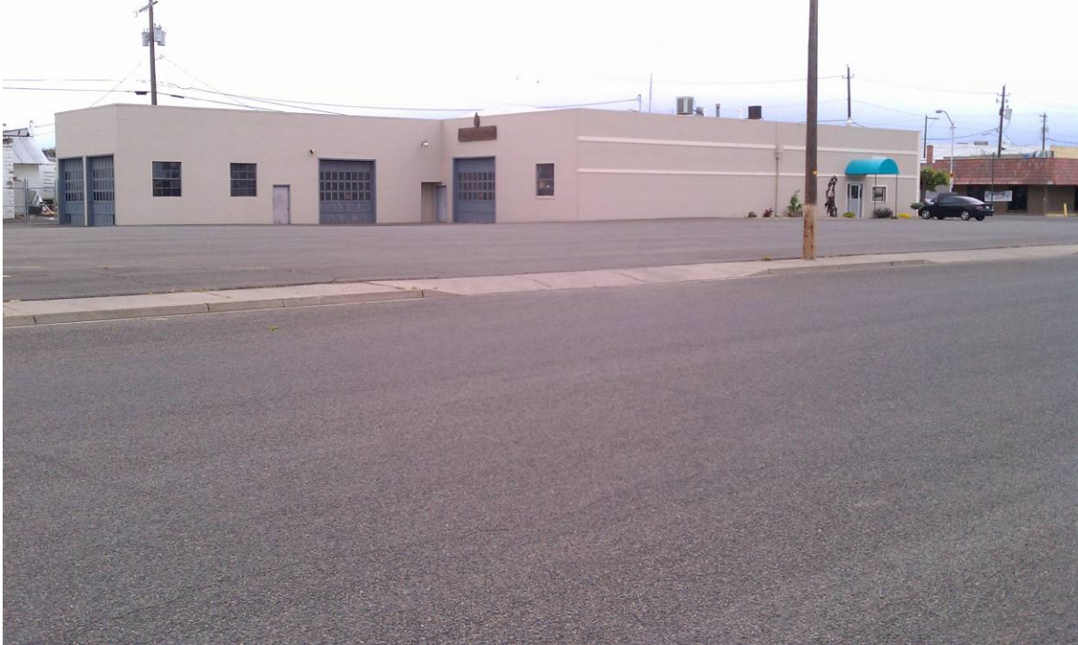
Photo 3: CNG Building and Parking Lot – from the northwest.
