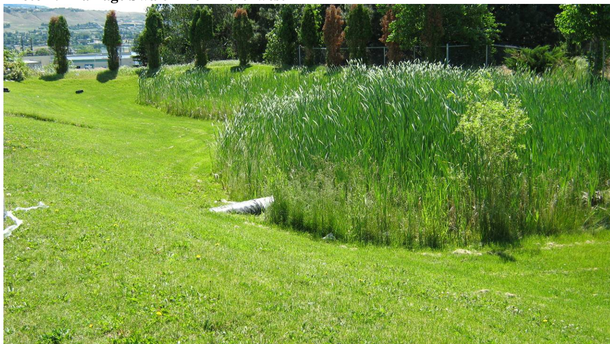
Photo 4: Drainage Swale - from northwest
