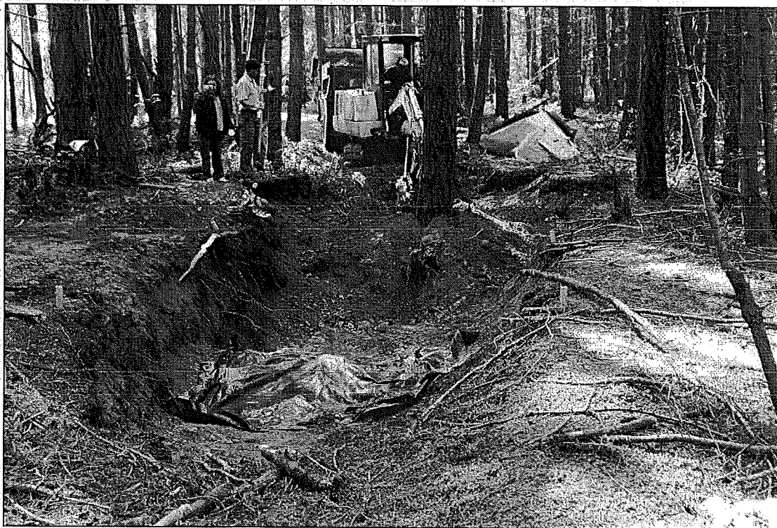
Photo 4: Completed trench excavation.
