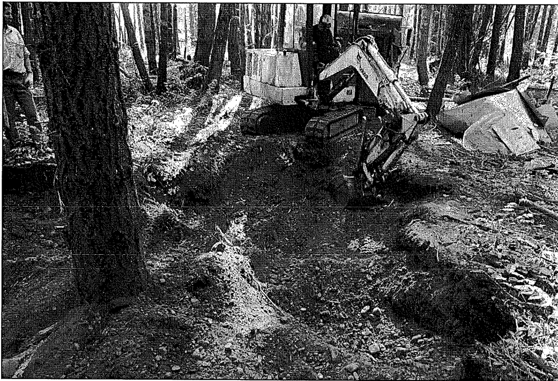
Photo 3: Western portion of trench excavation.
