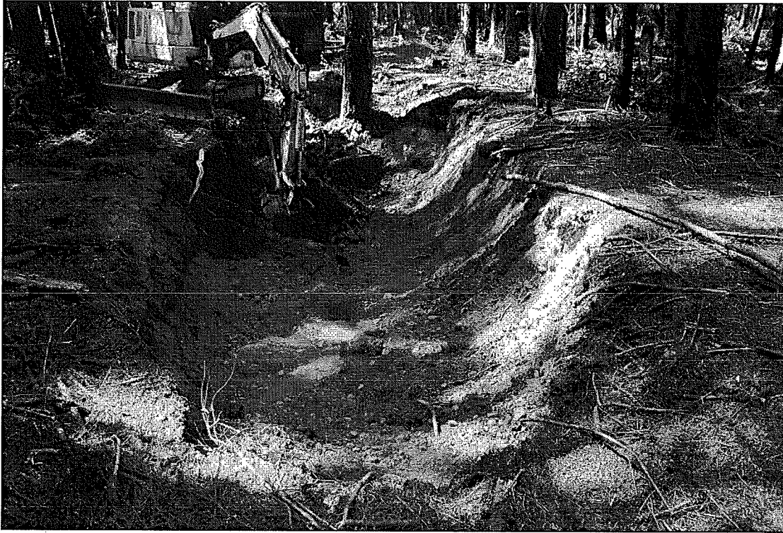
Photo 1: Eastern portion of trench excavation.
