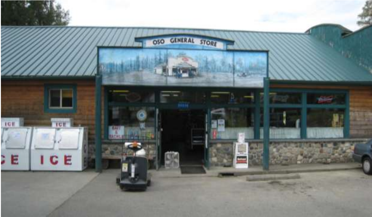
Photo 1: Front of store - from the east
