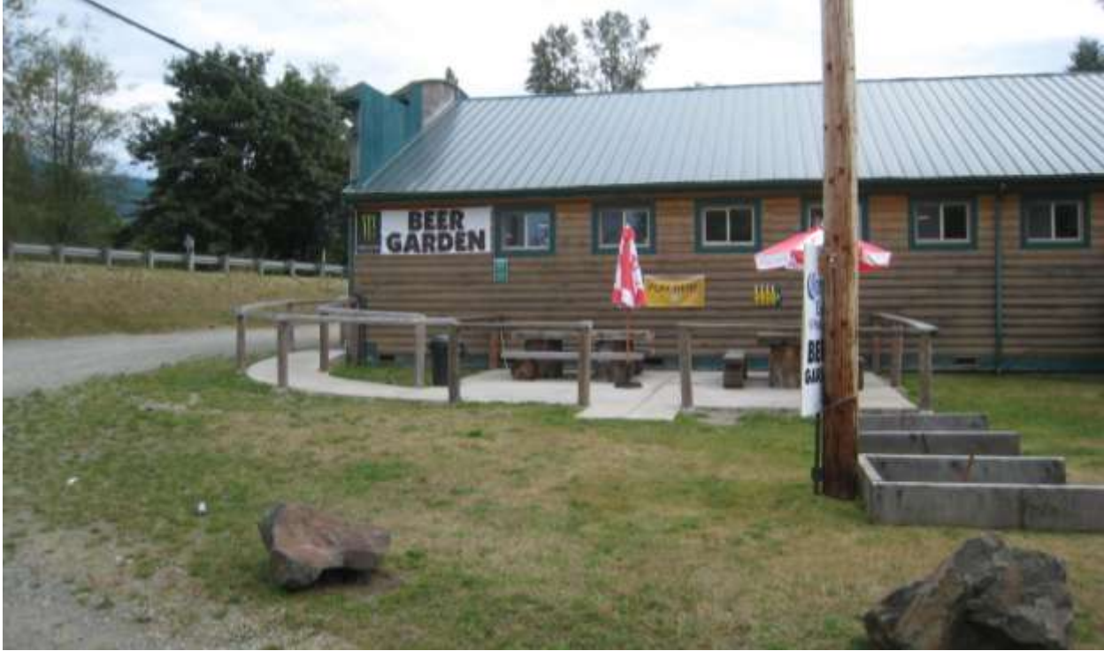
Photo 3: Rear of store building - from the west
