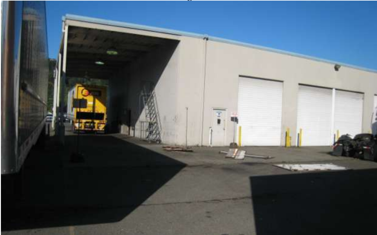
Photo 4: East side of the maintenance building
