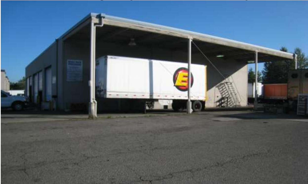
Photo 1: UST under concrete pad at right, south side of maintenance bldg.
