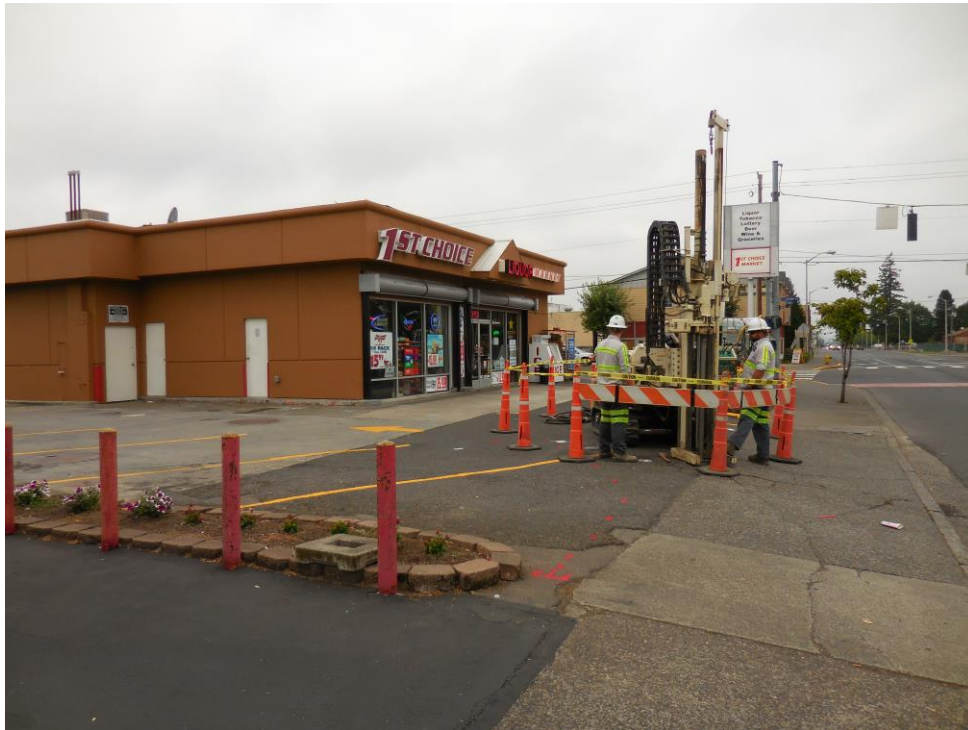
Photo 1 View looking west. Injecting ISCO into IP-01.
