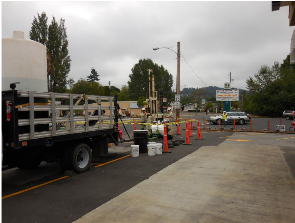
Photo 3 View looking east. Injecting ISCO into IP-01. Injection equipment in foreground.
