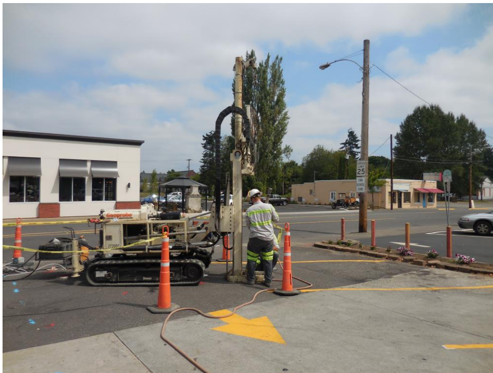
Photo 4 View looking north. Injecting ISCO into IP-02 and rinsing equipment.
