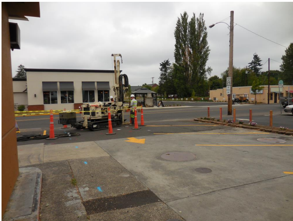
Photo 2 View looking north. Injecting ISCO into IP-01.
