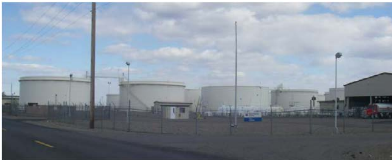
Antigua Chevron Pipe Line Company Pasco Bulk Terminal Site
