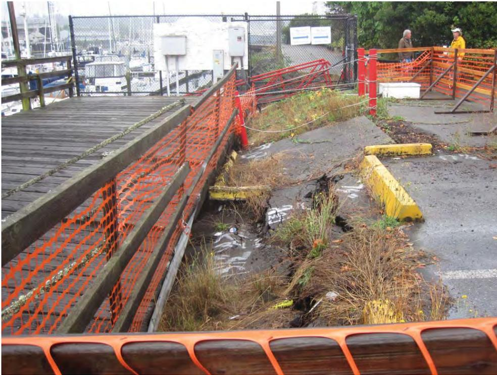
Photograph 1 – Settlement of the upland parking area resulting from bulkhead failure
