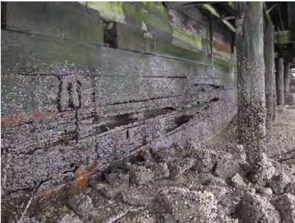
Photograph 4 – Deteriorated bulkhead wall
