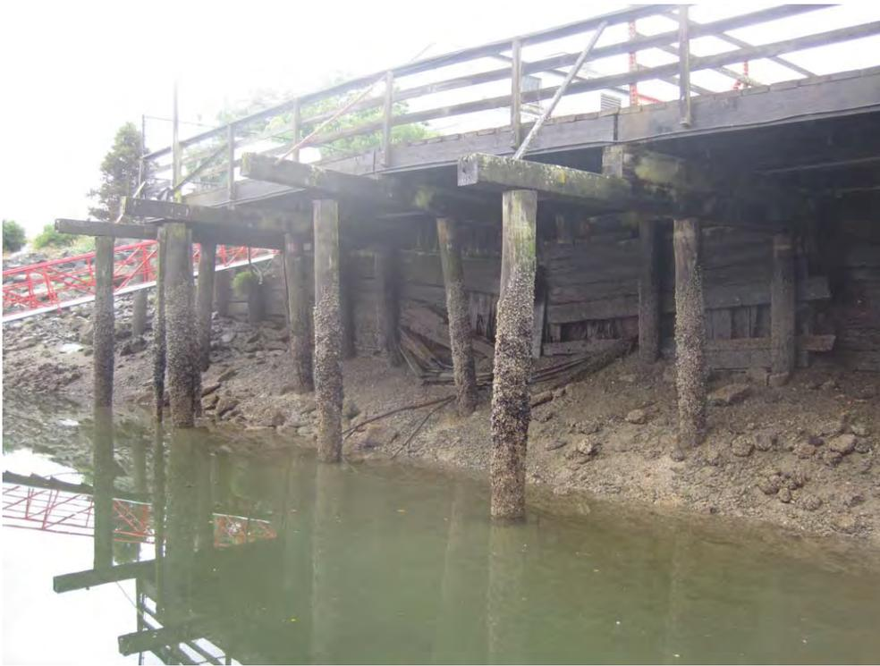
Photograph 3 – Bulkhead failure
