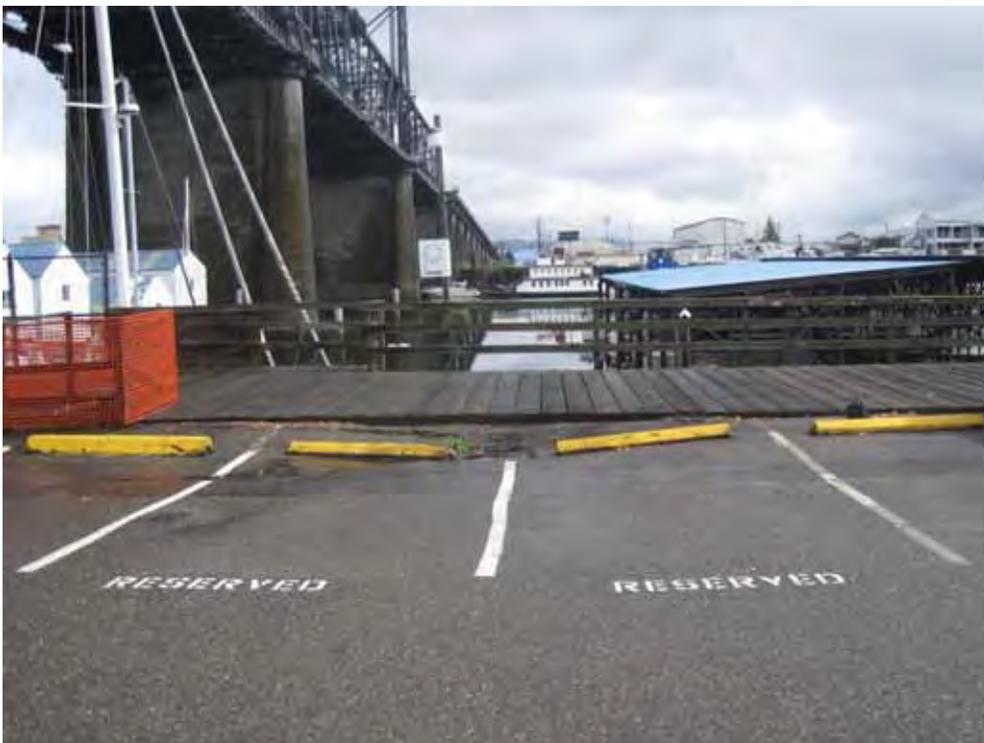
Photograph 2 – Settlement of the upland parking area resulting from bulkhead failure
