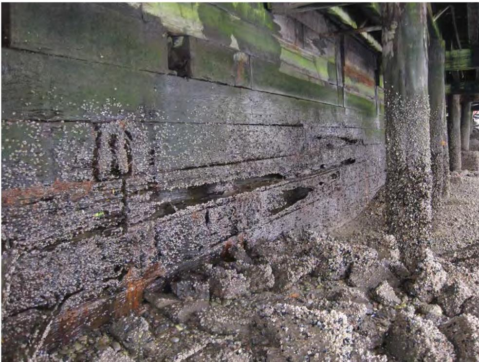
Photograph 4 – Deteriorated bulkhead wall
