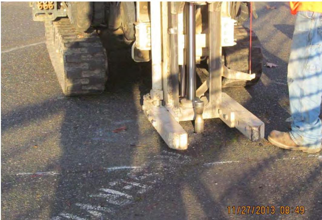
Photo 7. End of five foot core which may be retrieved, or stacked with a second five foot section.
