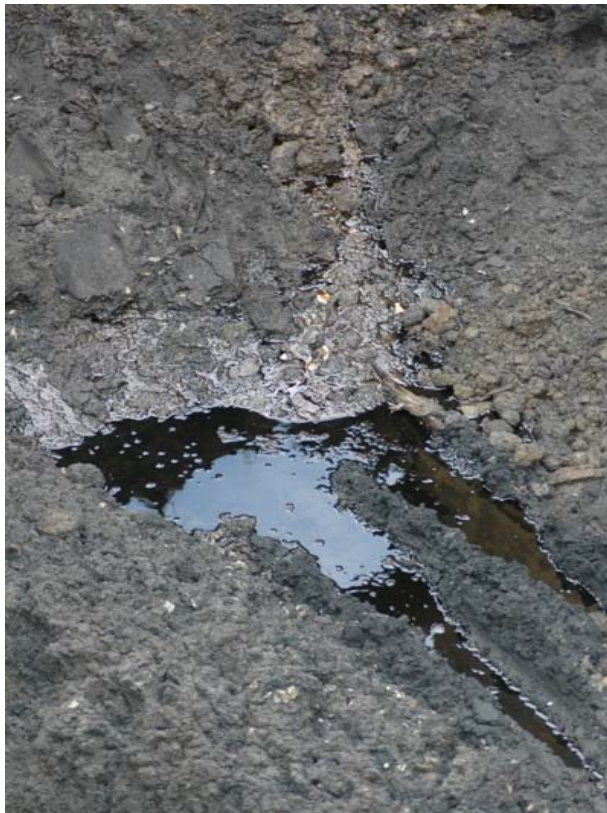
Photo 3. Oil and water entering sump excavation
