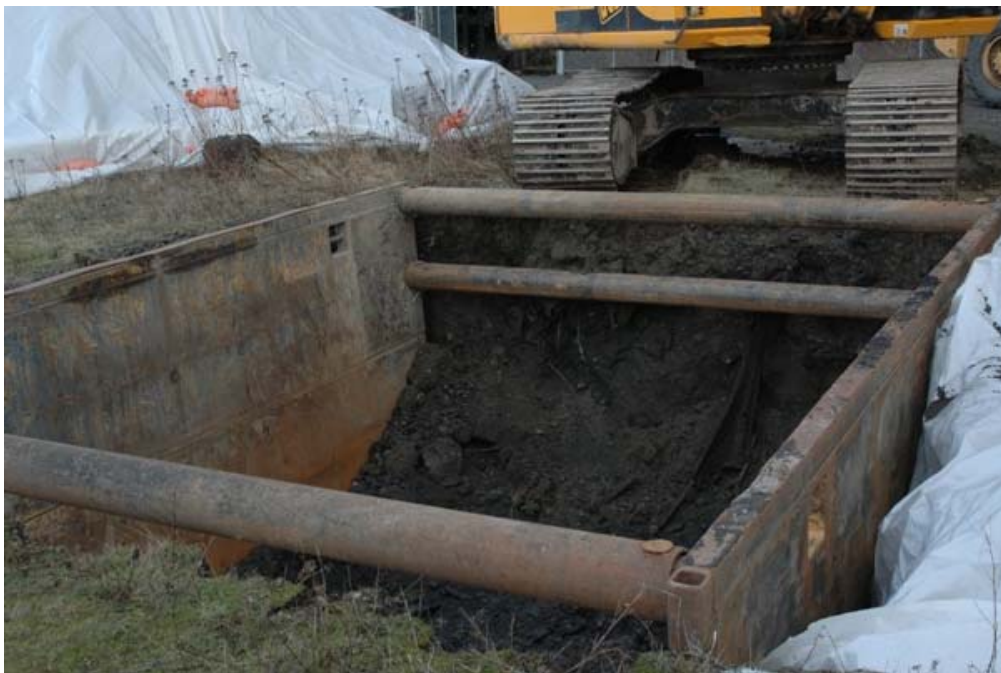
Photo 2. Trench box in place
