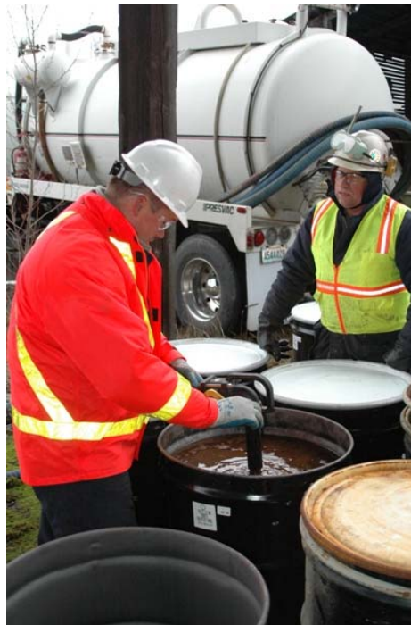
Photo 12. Transfer of recovered oil to drums
