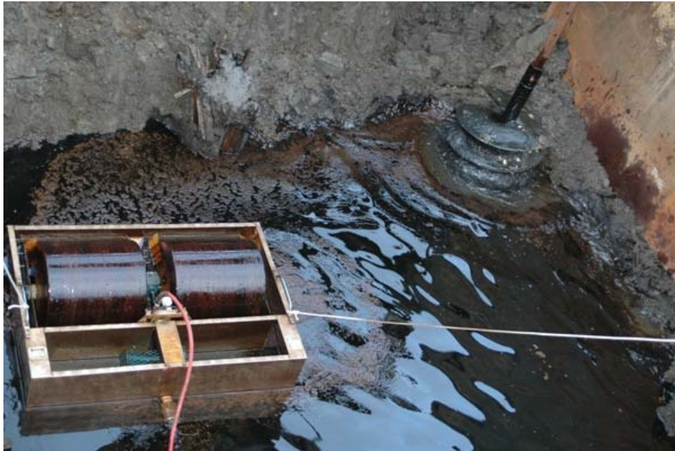
Photo 7. Soil agitation using helical auger, with simultaneous oil recovery
