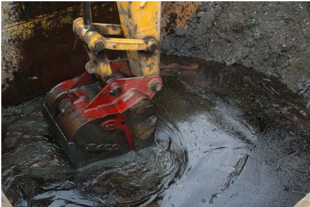
Photo 8. Soil agitation using excavator bucket
